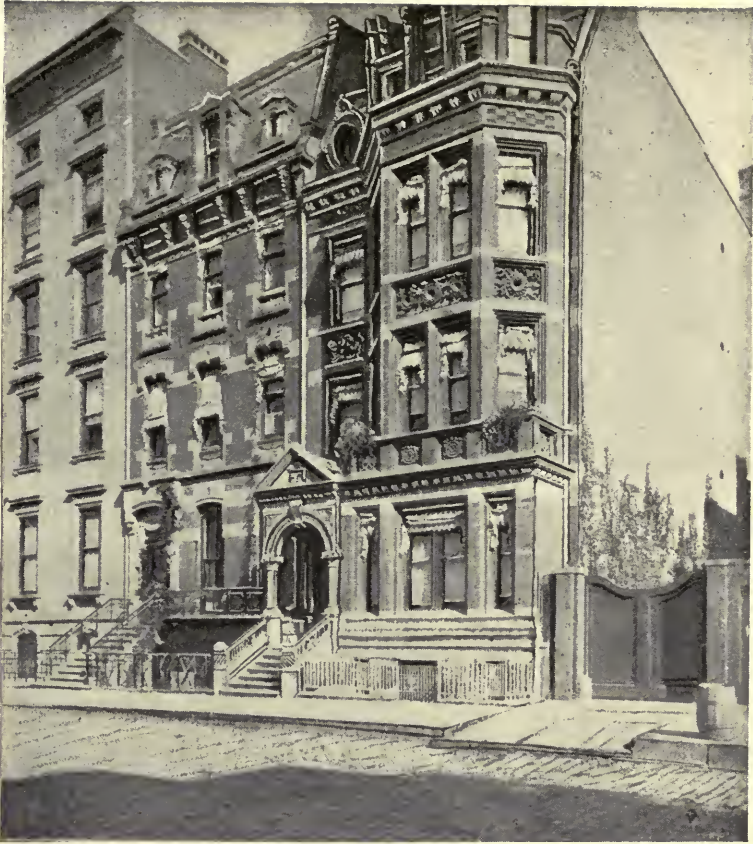
THE FIRST TERRA COTTA BUILDING ERECTED IN NEW YORK CITY.
