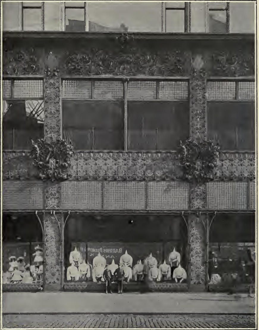
A General View of the Ornamental Iron Work of the Lower Stories. THE SCHLESINGER & MAYER BUILDING.
