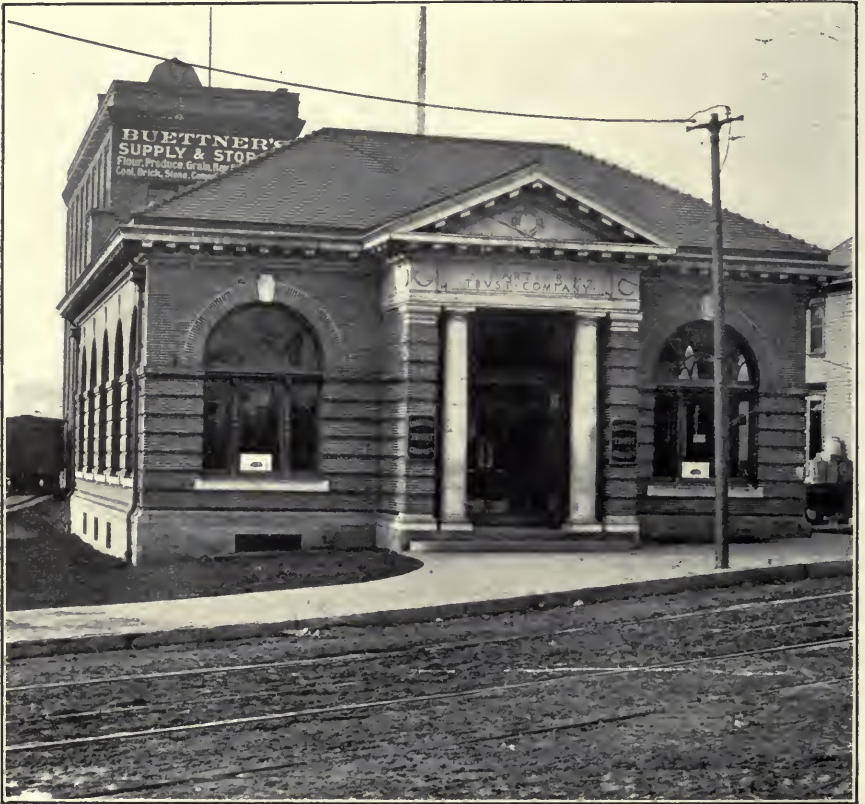
CHARTIERS TRUST CO. BUILDING.
