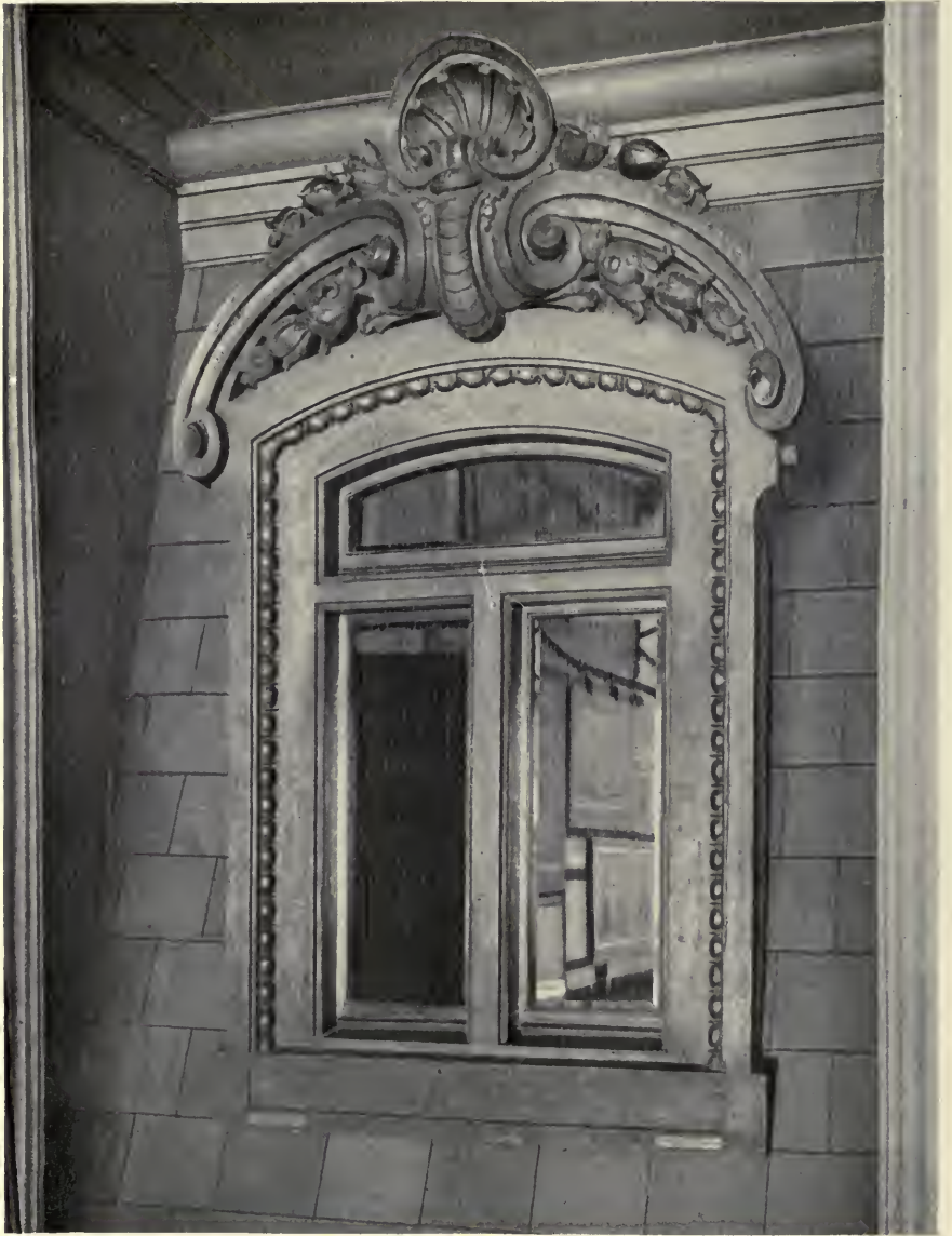
METALLIC WINDOW FRAME ON THE RESIDENCE OF SENATOR CLARK. Executed by the Henry-Bonnard Co. Lord & Hewlett, Washington Hull and K. M. Murchison, Associated.
