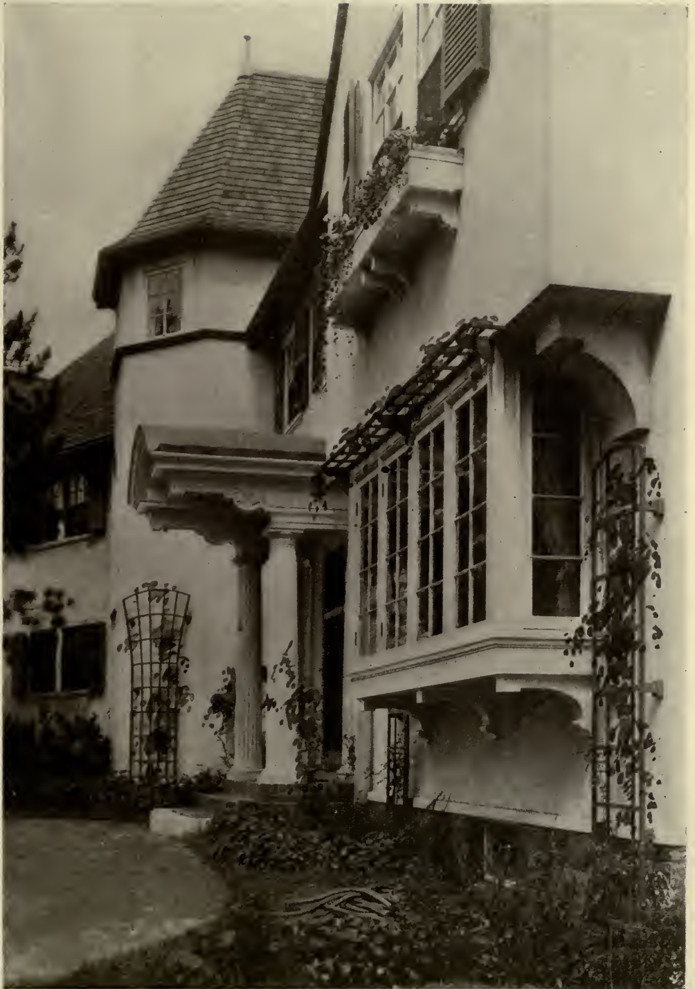
ENTRANCE DETAIL—THE RESIDENCE OF A. H. MARKS, ESQ. Marblehead, Mass. Andrews, Jacques & Rantoul, Architects.
