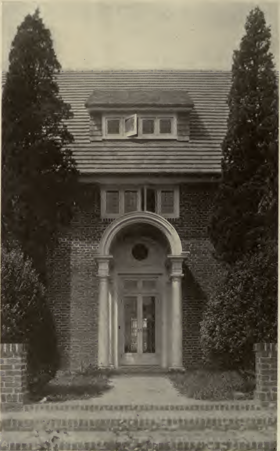
A HOUSE AT HEWLETT, LONG ISLAND. ALBRO AND LINDBERG, ARCHITECTS.
