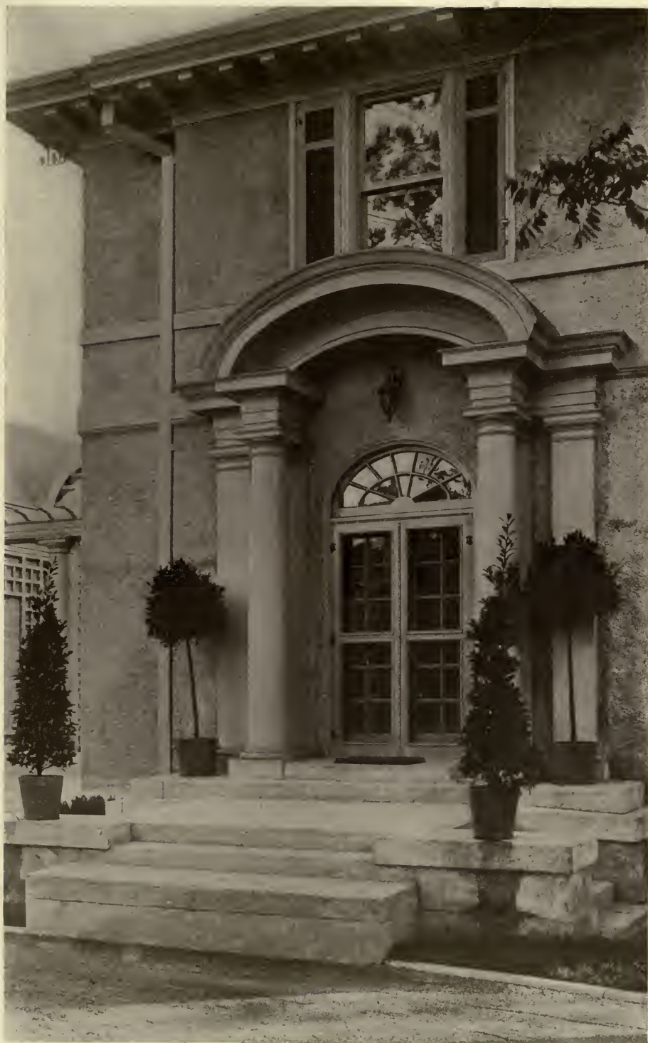
DETAIL OF ENTRANCE—RESIDENCE OF NELSON WHITNEY, ESQ. New Orleans, La. De Buys, Churchill & Labouisse, Architects.
