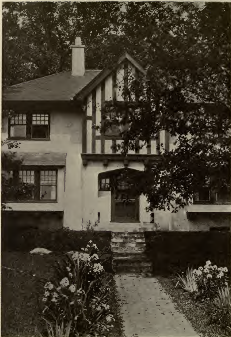
RESIDENCE OF MR. C. I. MARVIN, LAWRENCE PARK, W. Bronxville, N. Y. Wm. A. Bates, Architect.
