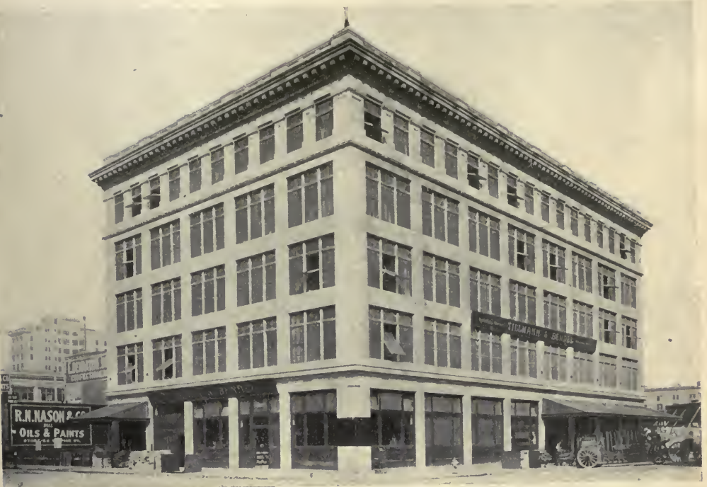
THE TILLMAN & BENDEL WAREHOUSE, SAN FRANCISCO, CAL. MacDonald & Applegarth, Archts.
