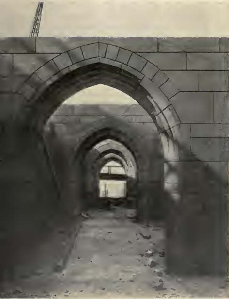
SOUTH TRIFORIUM LOOKING WEST.
