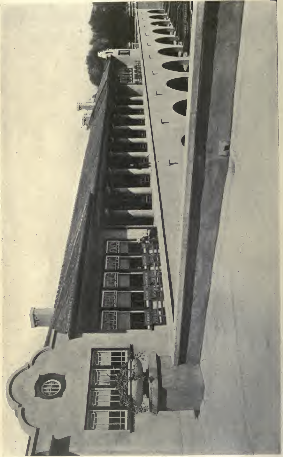
FIG. 2—SHOWING CONCRETE USED AS A WALL WITH ARCHED OPENINGS.
