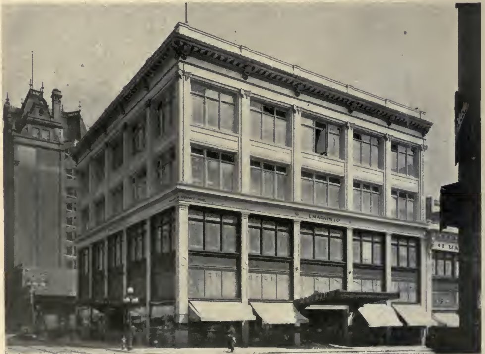
A RETAIL STORE—I. MAGNIN CO., SAN FRANCISCO, CAL. Wm. Mooser, Architect.
