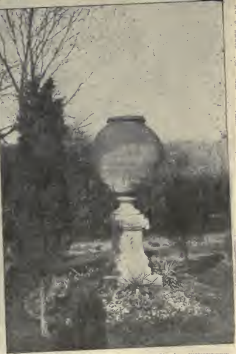
FIGS. 16, 17, 18 AND 19—CONCRETE USED FOR GARDEN ORNAMENT.
