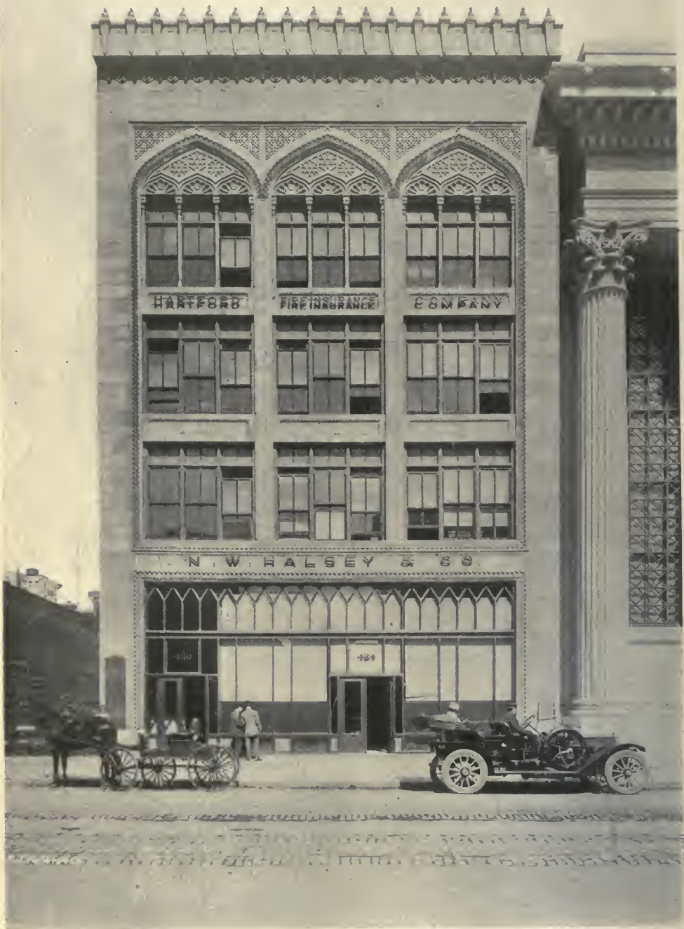
THE N. W. HALSEY & CO. BUILDING—CALIFORNIA STREET— SAN FRANCISCO, CAL. N. F. WOODRUFF, ARCHITECT.
