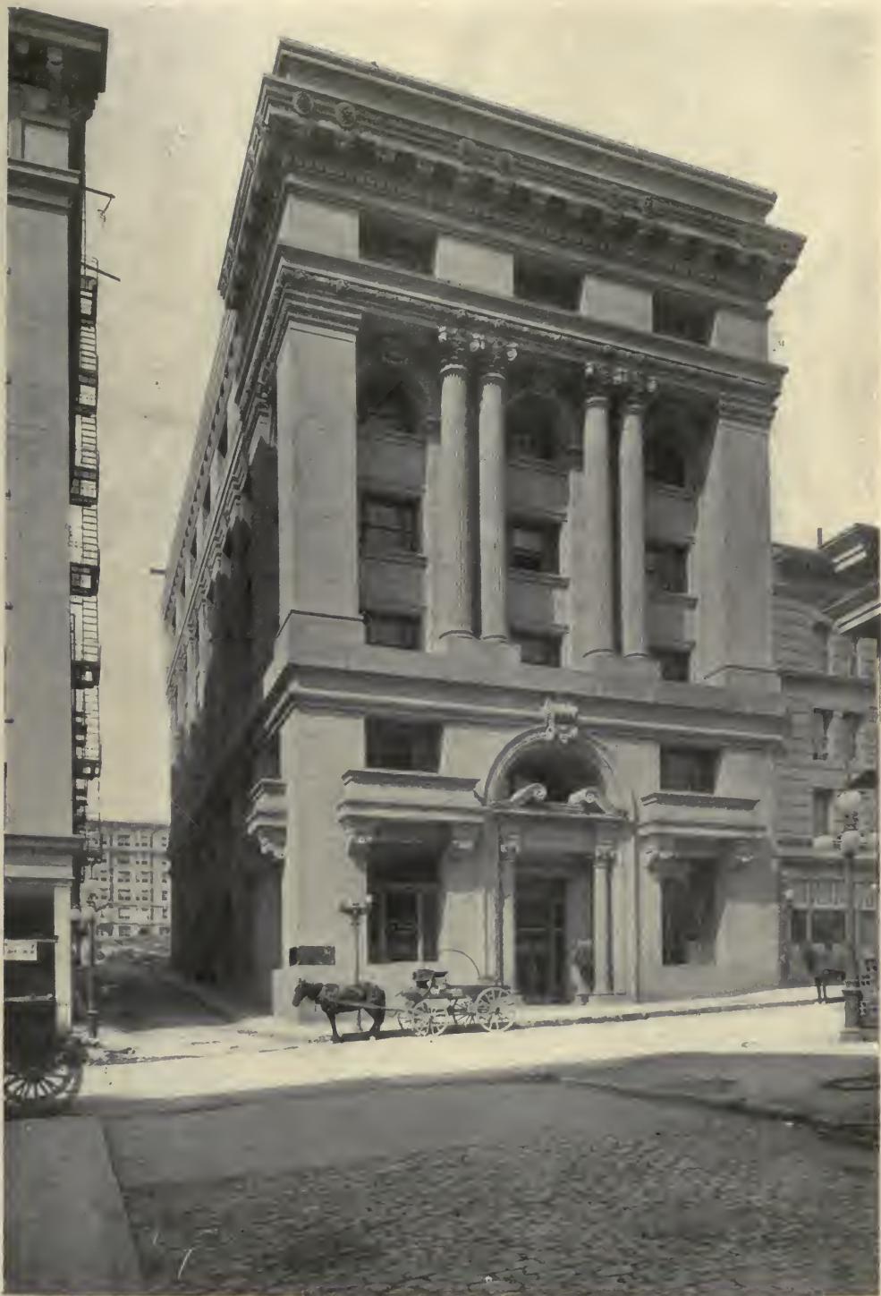
THE HOME TELEPHONE COMPANY BUILDING, SAN FRANCISCO, CALIFORNIA. COXHEAD & COXHEAD, ARCHITECTS.
