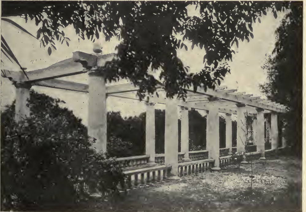
FIG. 4—DORIC COLUMNS OF MOULDED CONCRETE.
