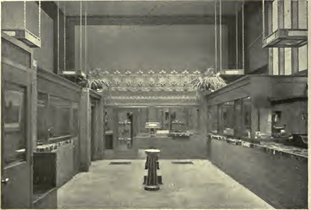
GENERAL INTERIOR VIEW LOOKING TOWARD VAULTS—MERCHANTS NATIONAL BANK, GRINNELL, IOWA. Louis H. Sullivan, Architect.
