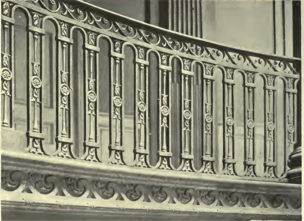
MARBLE BAND AT ROTUNDA. THIS CARVING HAD BEEN ALL BUT OBLITERATED BY PAINT— NEW YORK CITY HALL.
