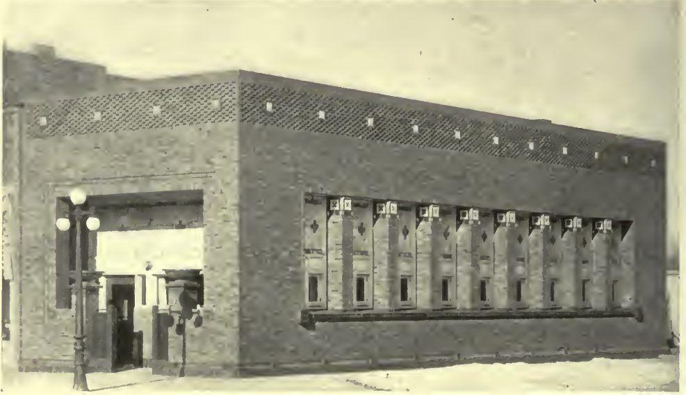
LAND AND LOAN OFFICE, ALGONA, IOWA. Louis H. Sullivan, Architect.
