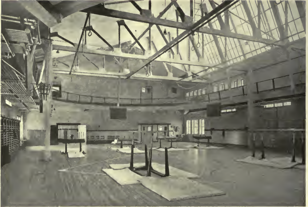
FIG. 17. MAIN GYMNASIUM ON THIRD FLOOR, CENTER SECTION, SHOWING ILLUMINATION THROUGH NORTH SKYLIGHT, THUS AVOIDING SHADOWS; STEEL TRUSSES FIREPROOFED WITH CONCRETE—Y. M. C. A. COLLEGE, CHICAGO.
