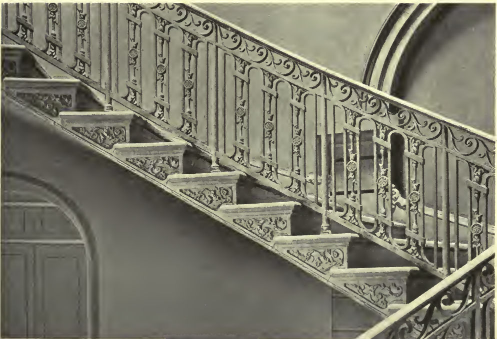
DETAIL OF MAIN STAIRWAY—NEW YORK CITY HALL.
