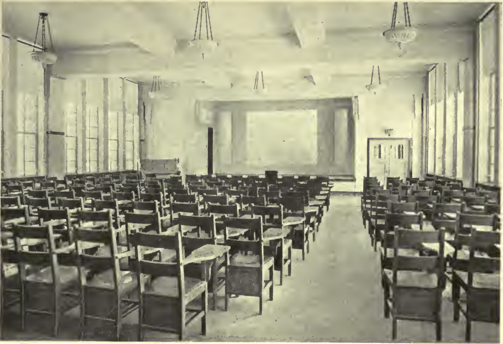
FIG. 15. CHAPEL AND SECTION ROOM ON SECOND FLOOR OF WEST SECTION, SHOWING REINFORCED CONCRETE GIRDERS IN CEILING WITH SPAN OF THIRTY-EIGHT FEET—Y. M. C. A. COLLEGE, CHICAGO.
