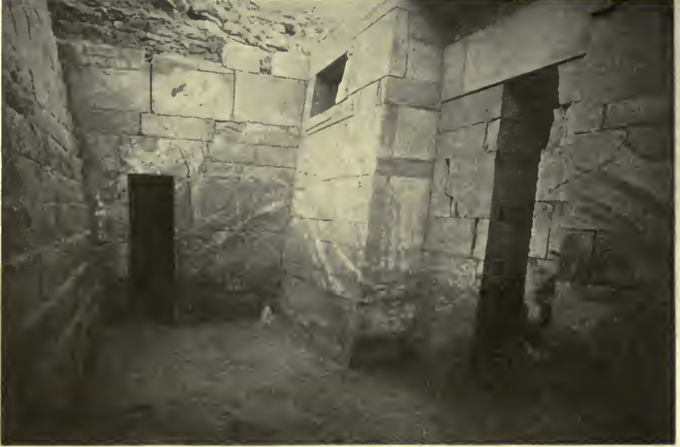
FIG. 4. TOMB OF PERNEB—VIEW OF COURTYARD, TOMB OF SHEPSESRE AT LEFT, DOOR TO SECONDARY OFFERING CHAMBER OPPOSITE, WINDOW LIGHTING STATUE CHAMBER TO RIGHT. PHOTOGRAPH MADE BEFORE REMOVAL TO THE METROPOLITAN MUSEUM.
