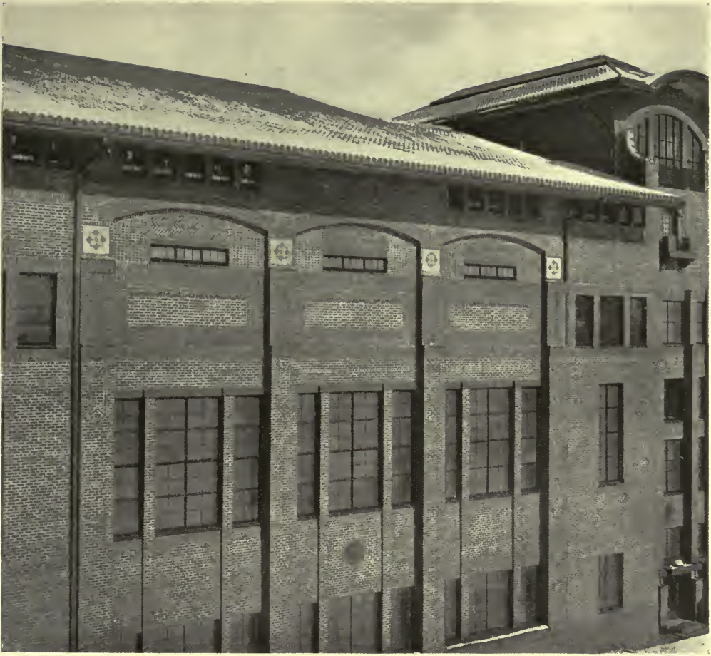
FIG. 6. CENTRAL, OR GYMNASIUM SECTION, FROM ROOF OF WEST WING—Y. M. C. A. COLLEGE, CHICAGO.
