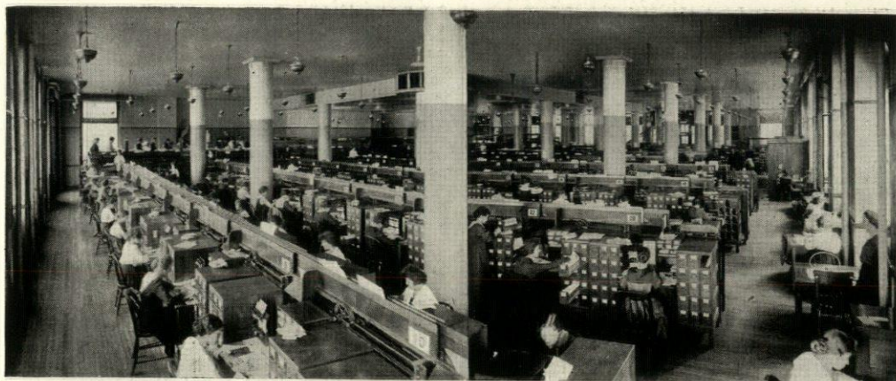
INDEX ROUTING DEPARTMENT—SEARS, ROEBUCK & CO'S PLANT, CHICAGO.
