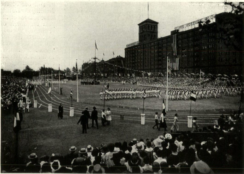
VIEW OF ATHLETIC FIELD IN FRONT OF THE MERCHANDISE BUILDING ON THE LAST FIELD DAY—SEARS, ROEBUCK & CO.'S PLANT, CHICAGO.
