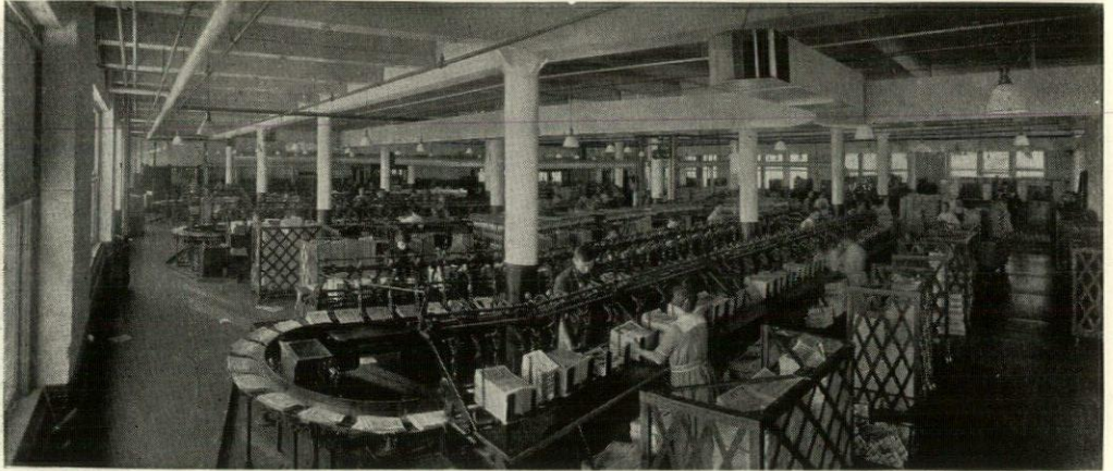
GATHERING AND BINDING MACHINES OF THE PRINTING DEPARTMENT—SEARS, ROEBUCK & CO.'S PLANT, CHICAGO.
