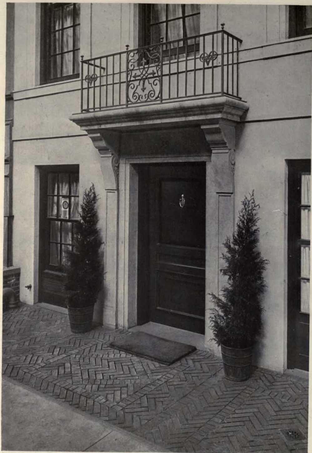
RESIDENCE OF GRENVILLE T. EMMET, ESQ., NEW YORK. MOTT B. SCHMIDT, ARCHITECT.
