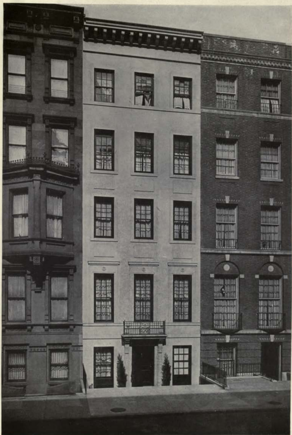
RESIDENCE OF GRENVILLE T. EMMET, ESQ., NEW YORK. MOTT B. SCHMIDT, ARCHITECT.
