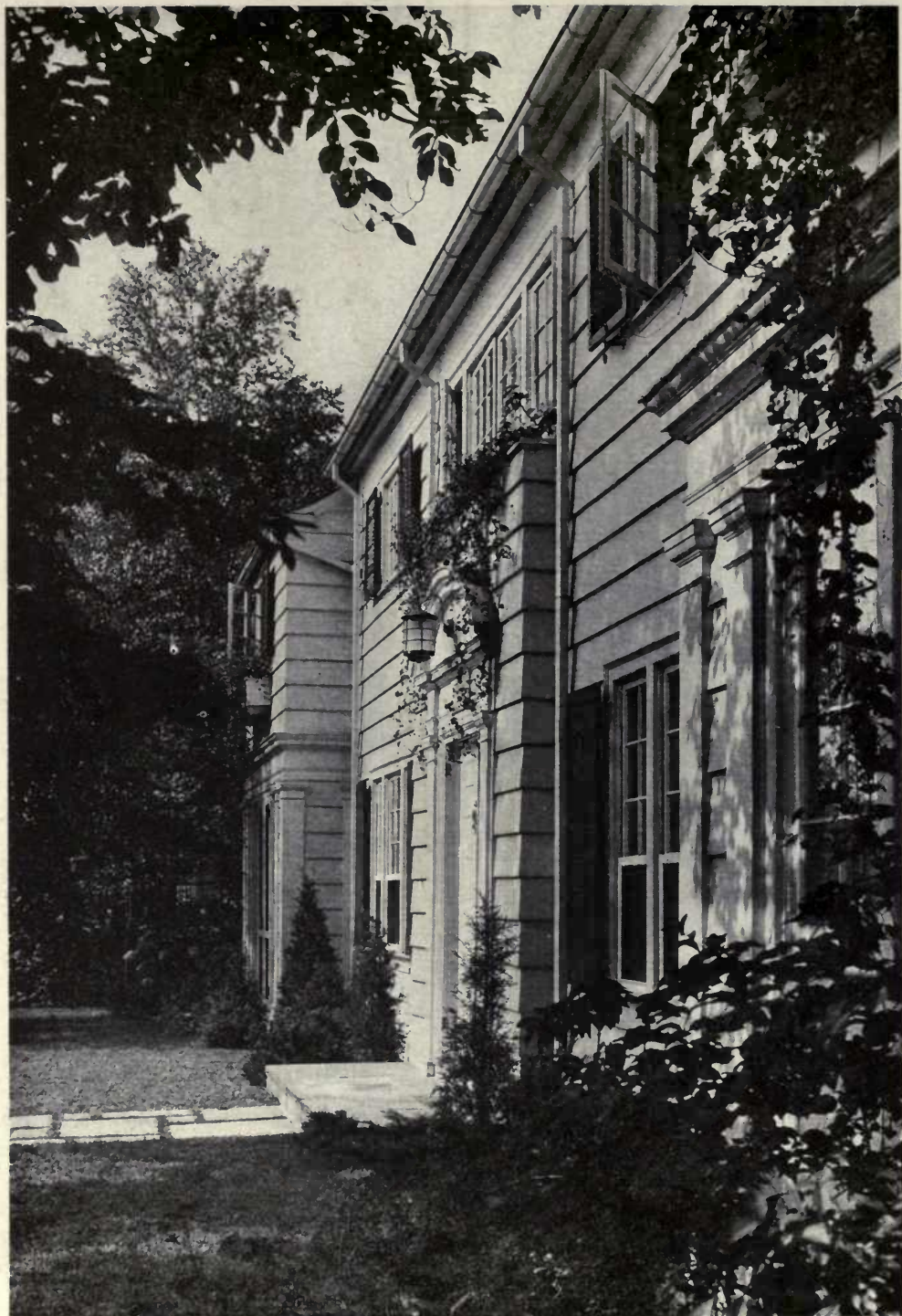
FIG. 2. DETAIL VIEW—RESIDENCE OF JOSEPH BUSH, ESQ., FIELDSTON, NEW YORK CITY. DWIGHT JAMES BAUM, ARCHITECT.
