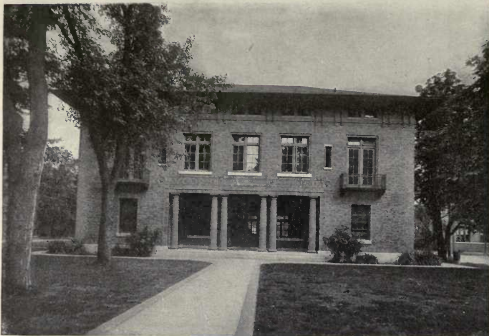
RECREATION BUILDING (CLARKE HALL), HAMPTON NORMAL AND AGRICULTURAL INSTITUTE, HAMPTON, VA. Ludlow & Peabody, Architects.
