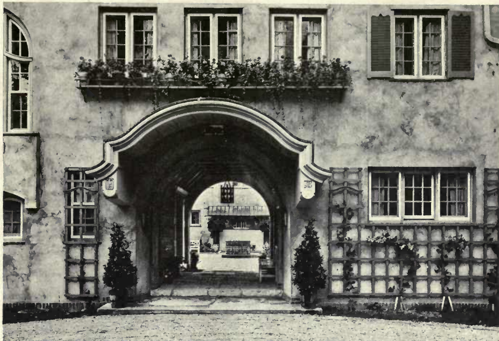
FIG. 13A. ENTRANCE TO COURT—RESIDENCE OF C. A. BARTLETT, ESQ., LAKE GENEVA, WIS. Howard Shaw, Architect.
