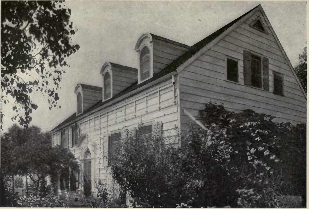
FIG. 95. EAST END—RESIDENCE OF EDWARD C. GUDE, ESQ., WHITE PLAINS, N. Y. William Lawrence Bottomley, Architect.
