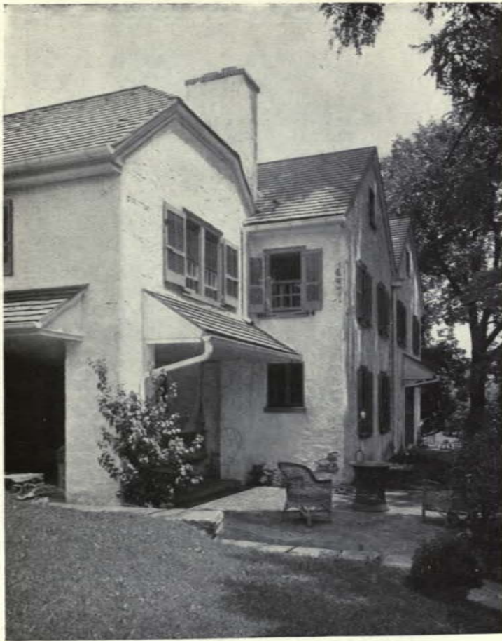
FIG. 58. TERRACE AND SOUTH FRONT—RESIDENCE OF MRS. ALBERT B. KELLEY, RADNOR, PA. Wilson Eyre & McIlvaine, Architects.
