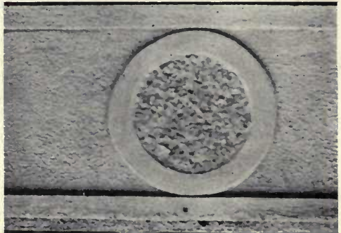
Interior of Circle Is Pebble Dash; Rim of Circle Troweled and Body Surface Sand-Floated.
