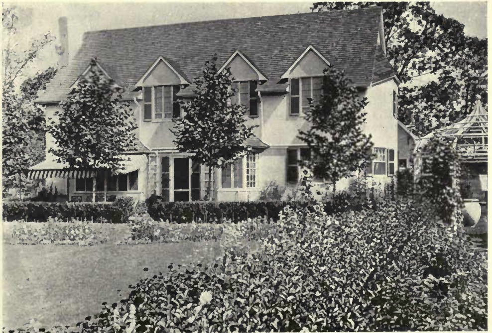
RESIDENCE OF FRANK A. COLBY, ESQ., HARTSDALE, N. Y. Architect and Owner.
