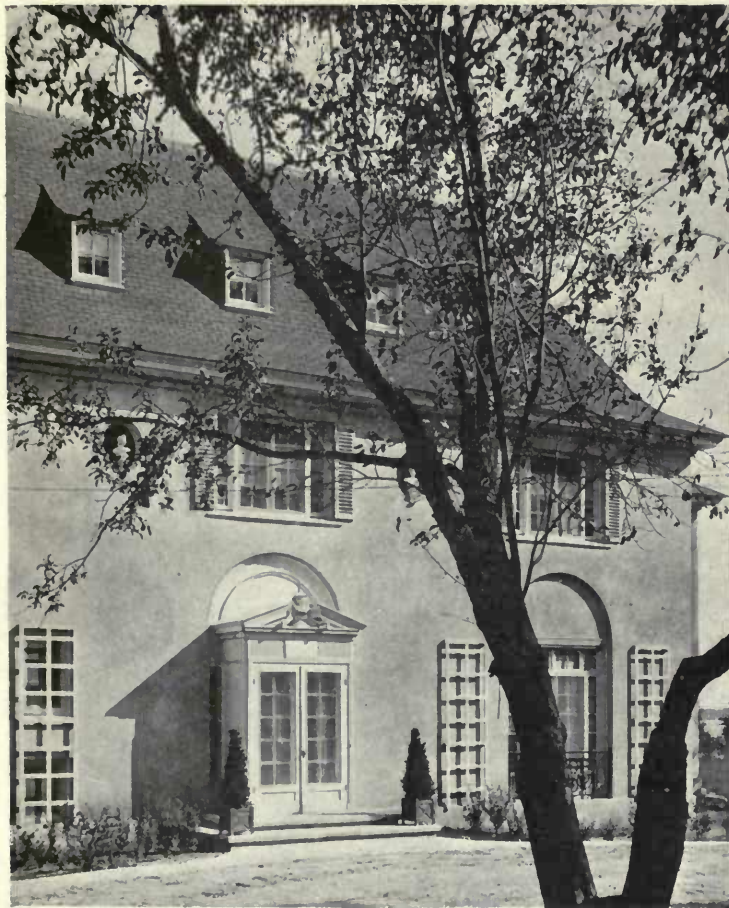
FIG. 107. MAIN ENTRANCE—RESIDENCE OF G. S. GAYLORD, ESQ., NEENAH, WIS. Childs & Smith, Architects.
