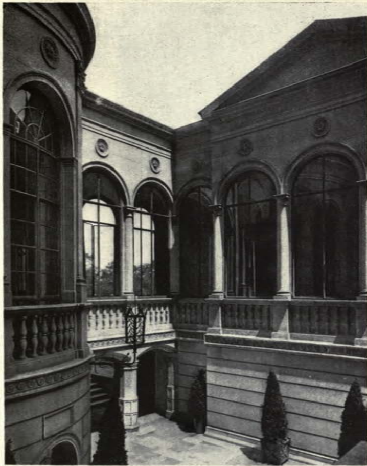
INNER COURT FROM SOUTHEAST CORNER—RESIDENCE OF OTTO H. KAHN, ESQ., NEW YORK. J. Armstrong Stenhouse, Architect.
