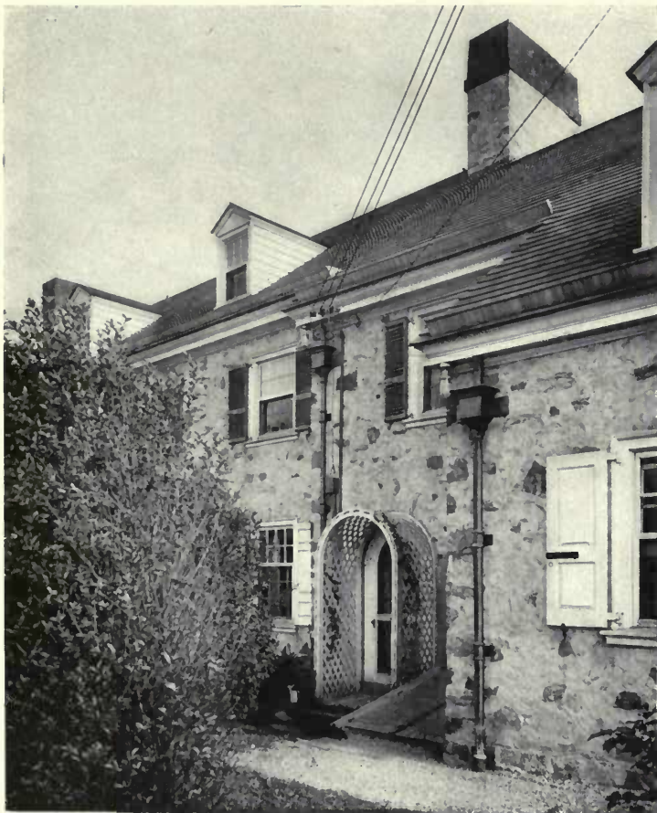
FIG. 54. DOOR TO MASTER'S ROOM—RESIDENCE OF E. H. FITCH, ESQ., MEADOWBROOK, PA. Tilden & Register, Architects.
