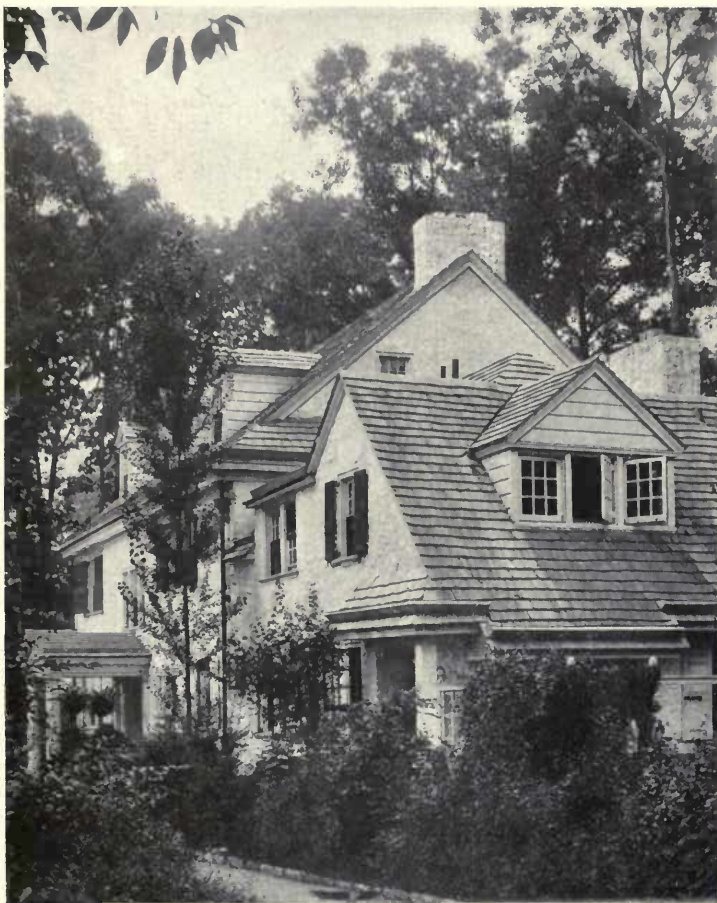
FIG. 49. SERVICE END—RESIDENCE OF C. E. MCINNES, ESQ., RYDAL, PA. Duhring, Okie & Ziegler, Architects.
