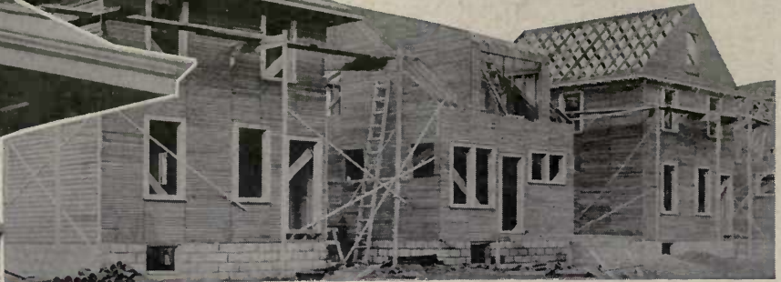
60 employees' residences, F. C. Mesa (Munitions), Irvington, N. J. Bishopric Sheathing used. Strombach and Mertens, Engineers and Architects.
