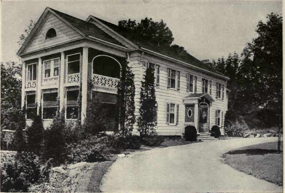
RESIDENCE OF WALTER M. BENNETT, ESQ., GREENWICH, CONN. Theodore E. Blake, Architect.
