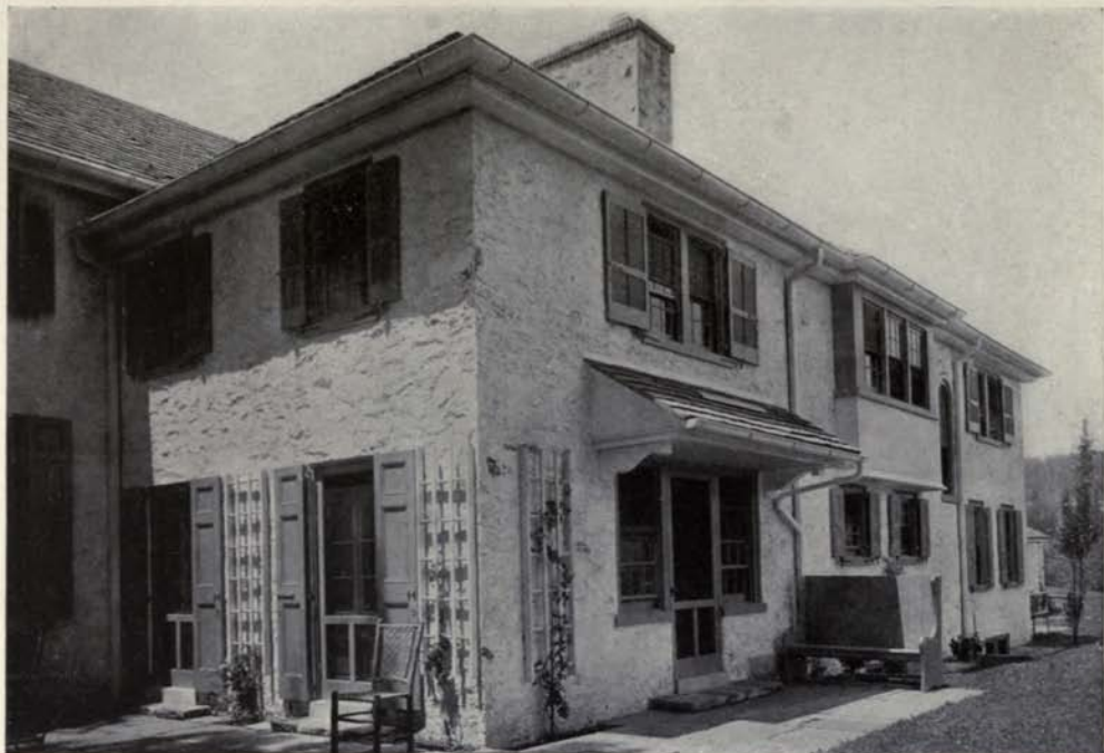
FIG. 60. BREAKFAST TERRACE AND EAST FRONT—RESIDENCE OF MRS. ALBERT B. KELLEY, RADNOR, PA. Wilson Eyre & McIlvaine, Architects.
