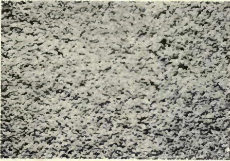
An Over-Coat Finish Called Rough-Casting, Which Gives the Coarsest Texture.
