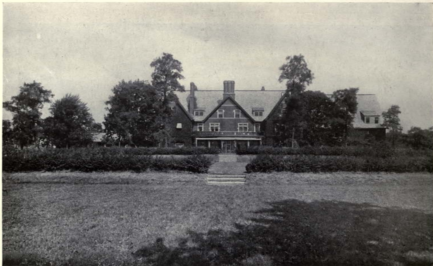
FIG. 20. RESIDENCE OF J. WATSON WEBB, ESQ., WOODBURY, L. L. CROSS & CROSS, ARCHITECTS.
