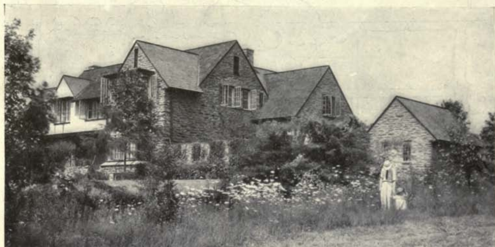
VIEW FROM EAST—RESIDENCE OF LEONARD T. BEALE, ESQ., ST. DAVIDS, PA. Mellor & Meigs, Architects.
