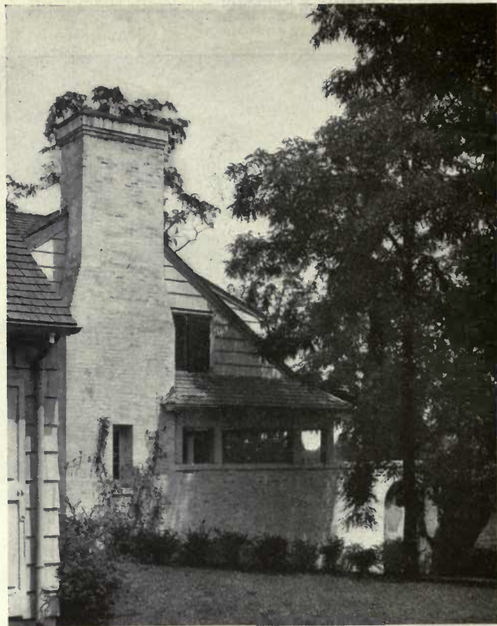
FIG. 40. KITCHEN WING—RESIDENCE OF H. P. WHITNEY, ESQ., GLEN COVE, L. I. Charles Willing of Furness, Evans & Co., Architect.
