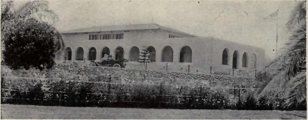
SCRIPPS PLAYGROUND BUILDING, LA JOLLA, CAL. Irving J. & Louis J. Gill, Architects.
