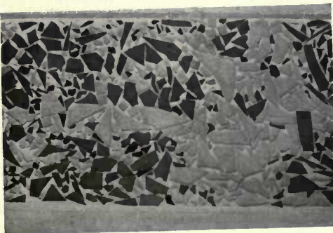
Mosaic Inlay With Glass of Various Colors. The Surface Is Plane, White Cement Filling the Crevices Between the Pieces of Glass.
