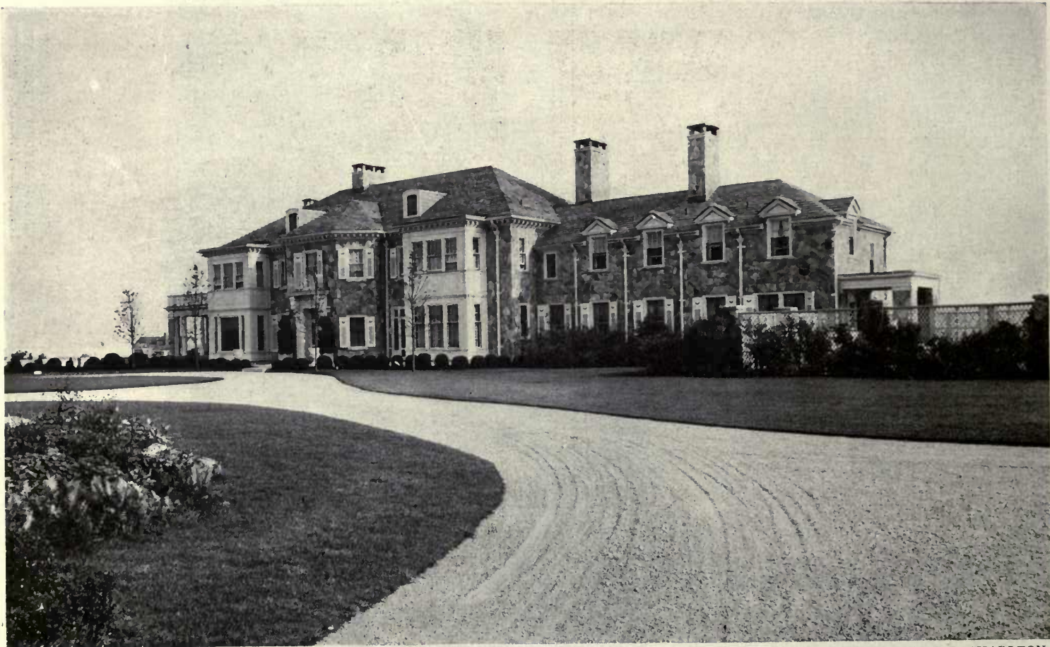
RESIDENCE OF EARLE P. CHARLTON, ESQ., WESTPORT HARBOR, MASS. FARLEY & HOOPER, ARCHITECTS.
