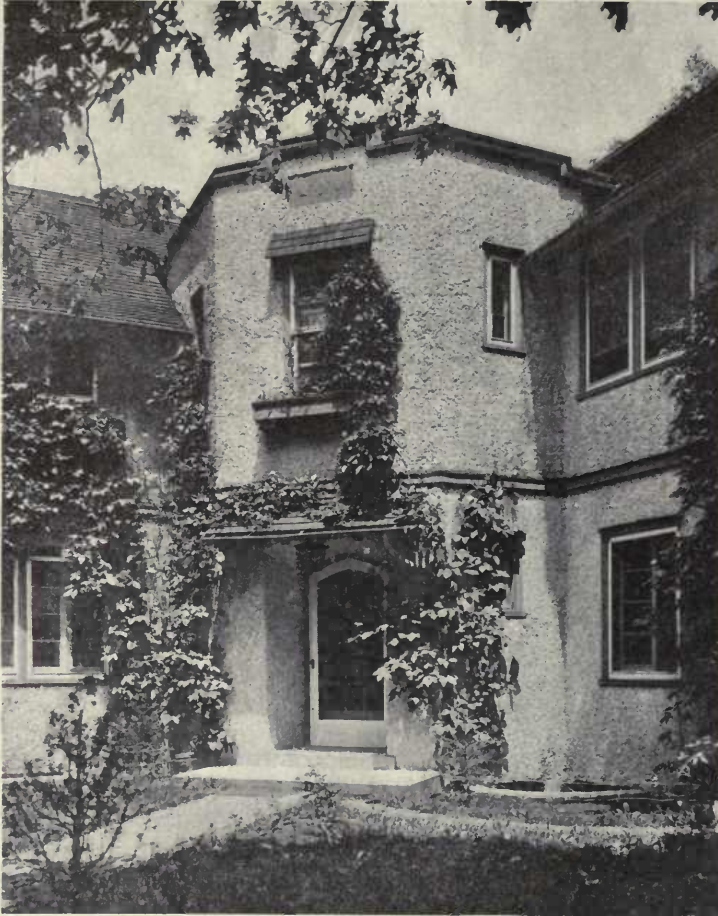
FIG. 102. RESIDENCE OF I. HELLER, ESQ., CEDAR LAKE, WIS. Brust & Philipp, Architects.
