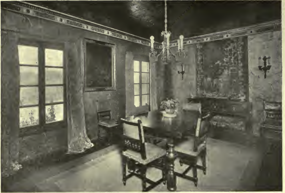
DINING ROOM—RESIDENCE OF JULIAN ELTINGE, ESQ., LOS ANGELES, CAL. Pierpont and Walter S. Davis, Architects.
