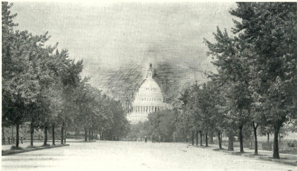
View east of the Capitol down Maryland Avenue—no planting in center, and a good view of the Dome
