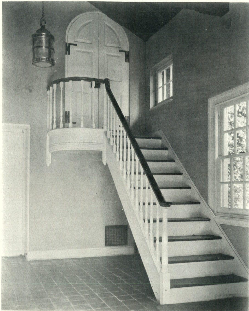
Interior of Porch CHRIST CHURCH, DOVER, DELAWARE. Frank R. Watson, George E. Edkins and William Heyl Thompson, Associated Architects
