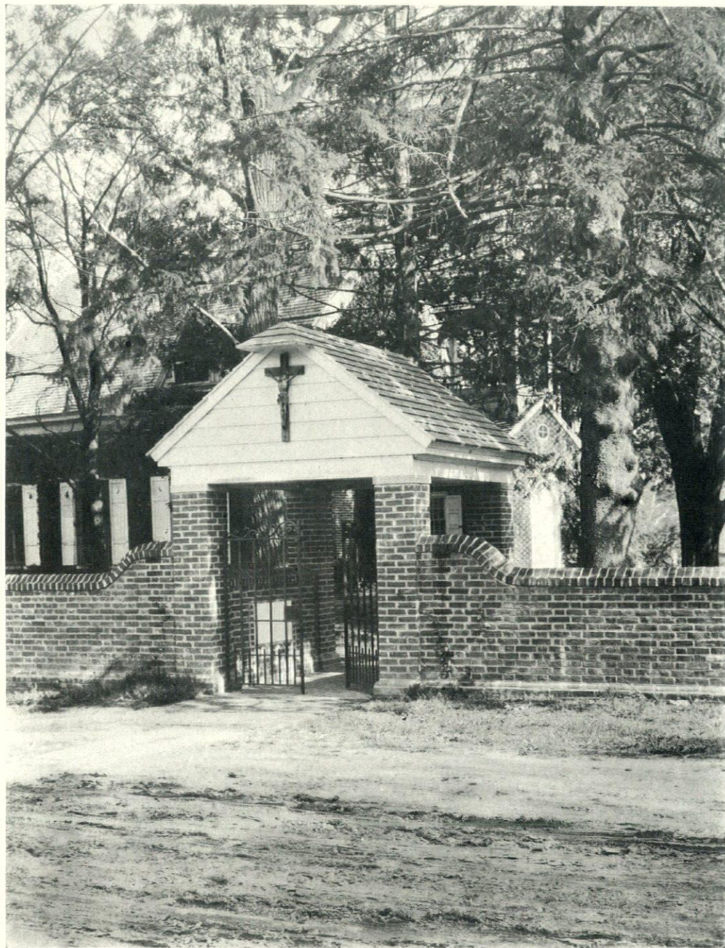
Lych Gate CHRIST CHURCH, DOVER, DELAWARE. Frank R. Watson, George E. Edkins and William Heyl Thompson, Associated Architects
