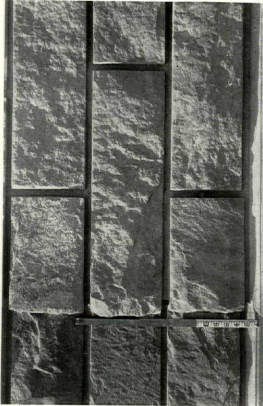
FIG. 10. WALL DETAIL, MODERN, PALACE IN VIA DEI SERVI, FLORENCE
