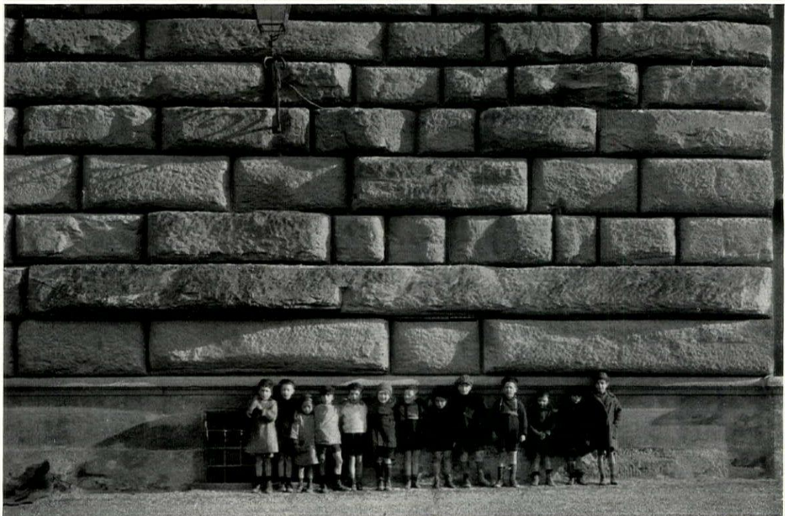
FIG. 41. MAIN FAÇADE. SHOWING TWENTY-SEVEN FOOT STONE, PITTI PALACE, FLORENCE BRUNELLESCHI, ARCHITECT, 1440 ITALIAN STONEMWORK. PART II
