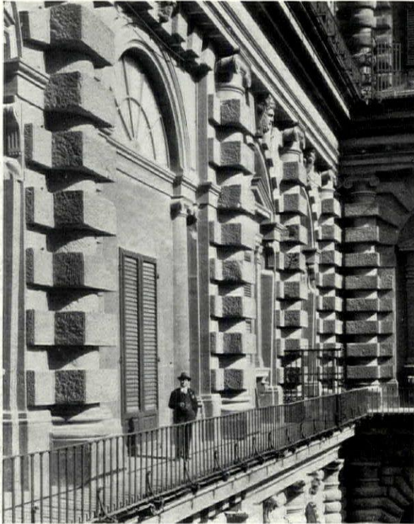
FIG. 35. ORDER AT SECOND FLOOR, GREAT COURT OF PITTI PALACE, FLORENCE AMMANATI, ARCHITECT, 1568
