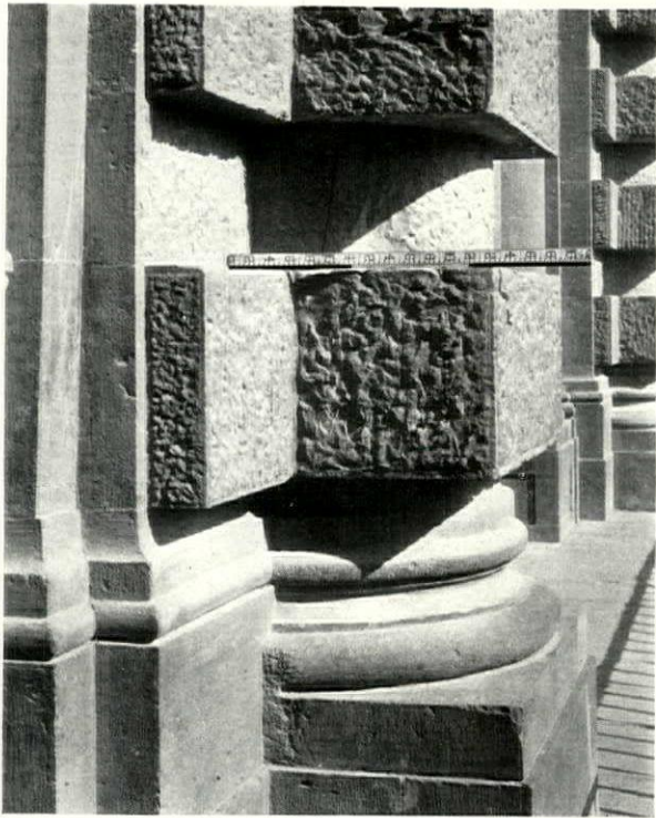
FIG. 31. PILASTER BASE AT SECOND FLOOR, GREAT COURT OF PITTI PALACE, FLORENCE AMMANATI, ARCHITECT, 1568
