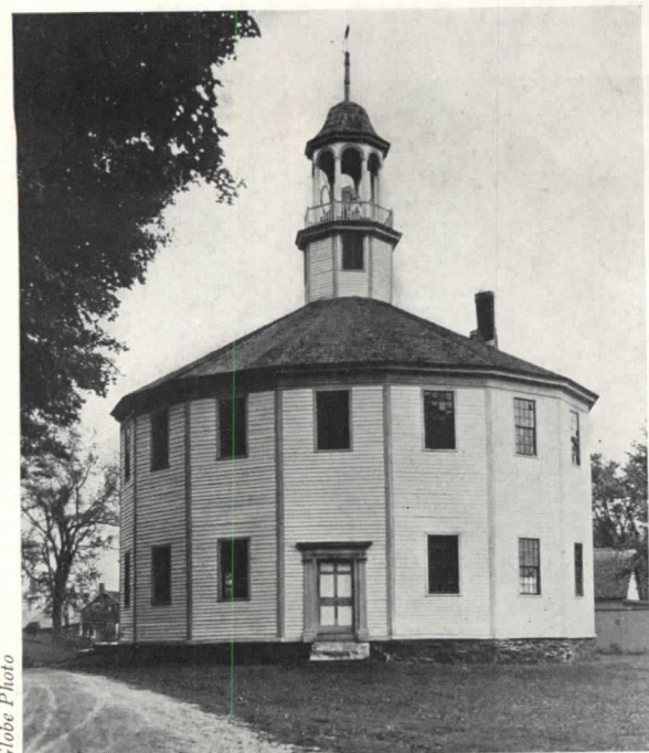
EARLY EXAMPLE OF THE DIVISION of labor is this 16-sided community church at Richmond, Vermont. Built in 1813 by 17 cooperative individuals, the 16-sided plan was hit upon as a means of dividing the work equally; the 17th built the cupola.
