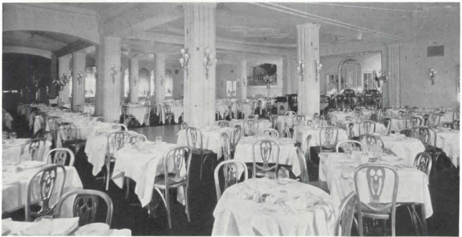
Hotel Belmont Plaza, New York City. Main dining room before modernization.
