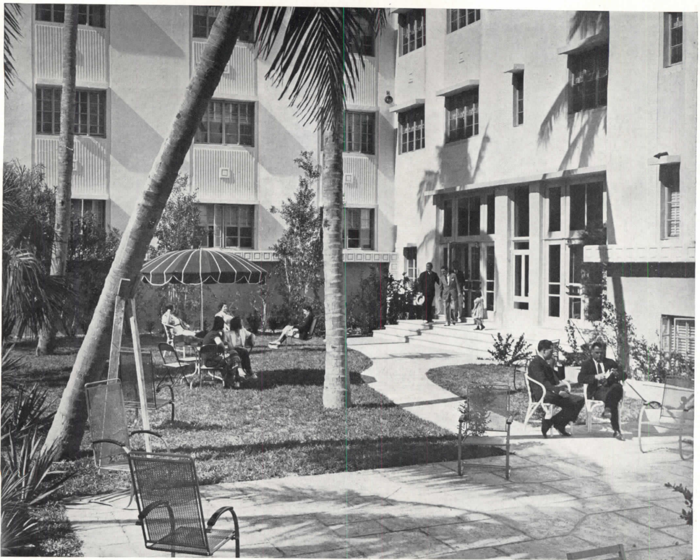
View of Patio and Lounge Entrance
