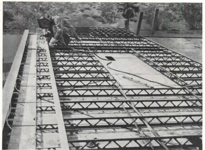
At left: Prefabricated bathroom, showing combined plumbing for bathroom, kitchen, and porch. Steel Craft House by Richard J. Neutra, Architect. Above, upper: Steel skeleton of standard parts, designed to resist lateral forces of earth shock and wind pressure. Richard J. Neutra, Architect. Above, lower: Expanded metal studs cut to length by torch, joined together by welding to produce strong and light building frame.
