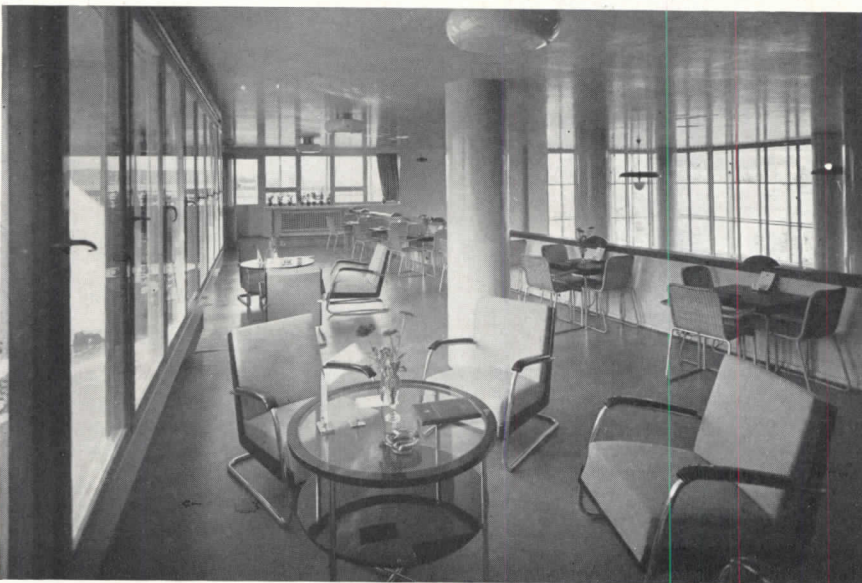
Balcony of Entrance Lobby
