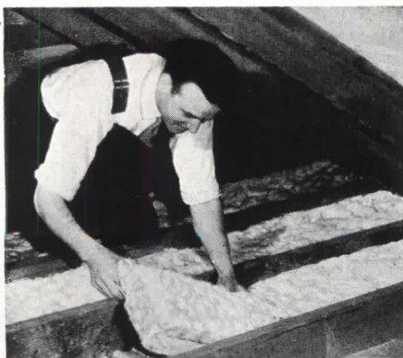
APPLYING Johns-Manville Ful-Thick Rock Wool Home Insulation in an open attic.
