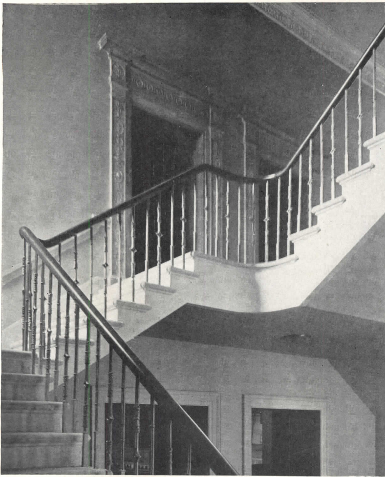
Main Stairway, rebuilt
