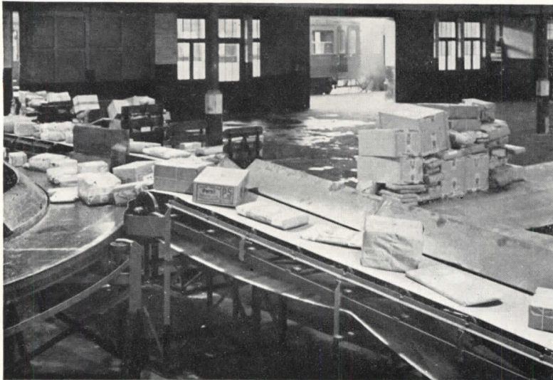
1. All incoming parcels are placed on a continuously moving conveyor . . .
