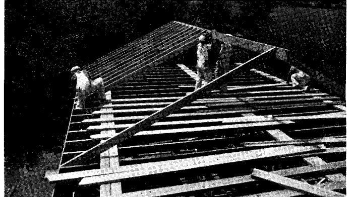
2 p.m. Nailing rafters; sheathing and shingles over.
