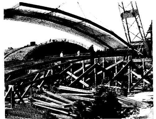
Section of arch reinforcing is picked up by crane for placing on arch centering.
