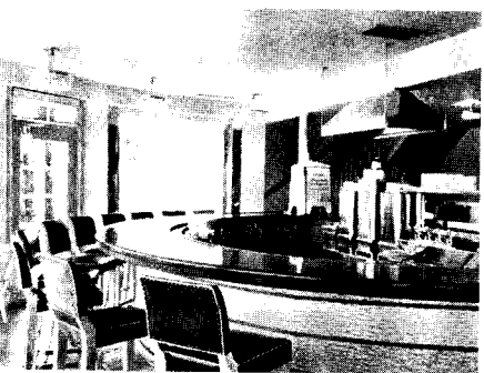
Exhaust over coffee urns, Carl's Viewpark Restaurant, Los Angeles; W. L. Schmolle, architect.
