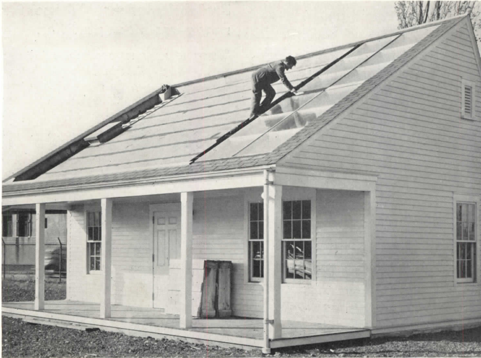
"Heat trap" in the roof of M.I.T.'s new experiment in conversion of solar energy. Note (upper left) the pyrheliometer, an instrument for recording sunlight intensities.
