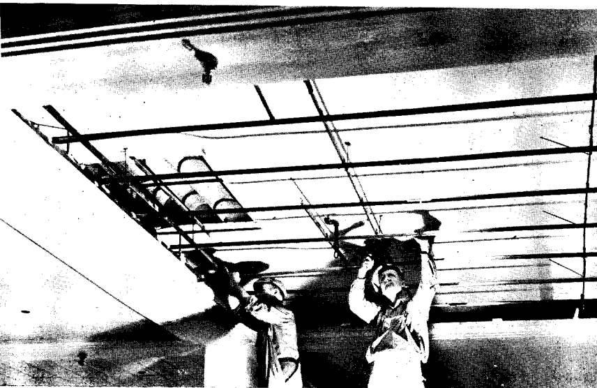
Integration of sound control and air conditioning: space between structural and suspended ceilings is a plenum; air passes through perforated-metal pans.
