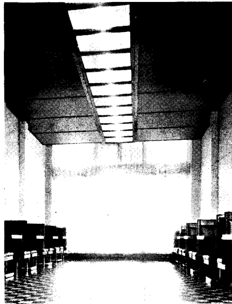
Diffused direct ceiling-panel lighting, Gotham Cafe, Hollywood, used as design motif; Richard Neutra, architect.
