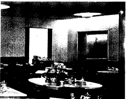
Combined air and lighting sources, Union Station, Kansas City; R. J. Raney-Holabird & Root, architects.
