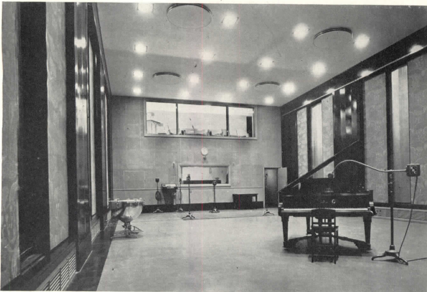
N.B.C. studio with sliding panels, rock wool with perforated metal over; V'd plaster between panels breaks up sound waves, preventing "flutter."
