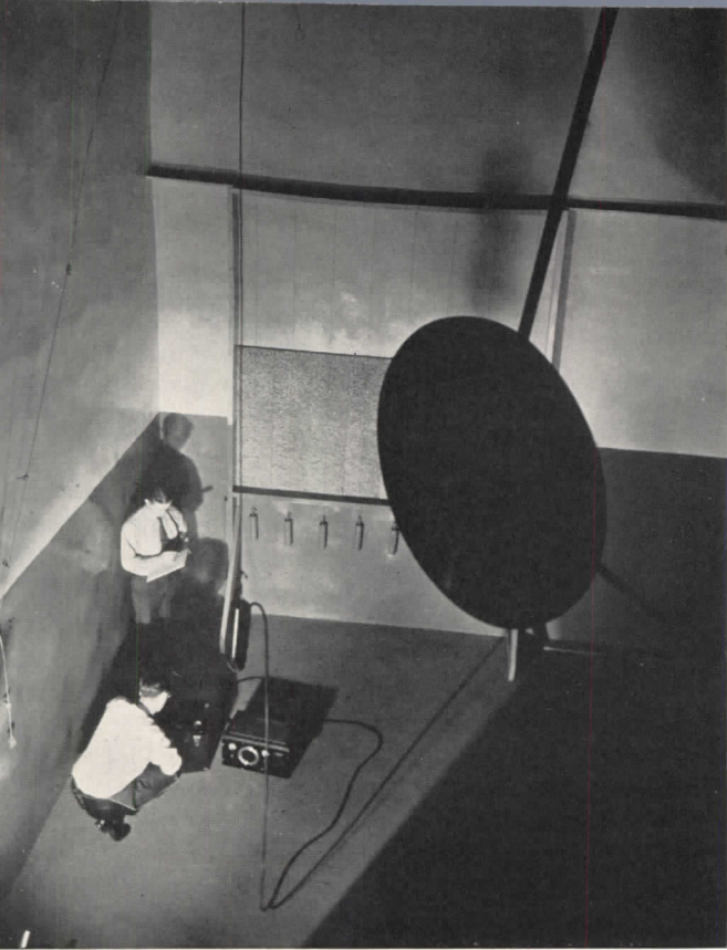
Reverberation chamber for measuring sound absorption
