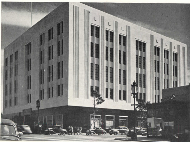
THIRTEEN VOTES: the I. Magnin Co. Department Store. Myron Hunt and H. C. Chambers were the architects.
