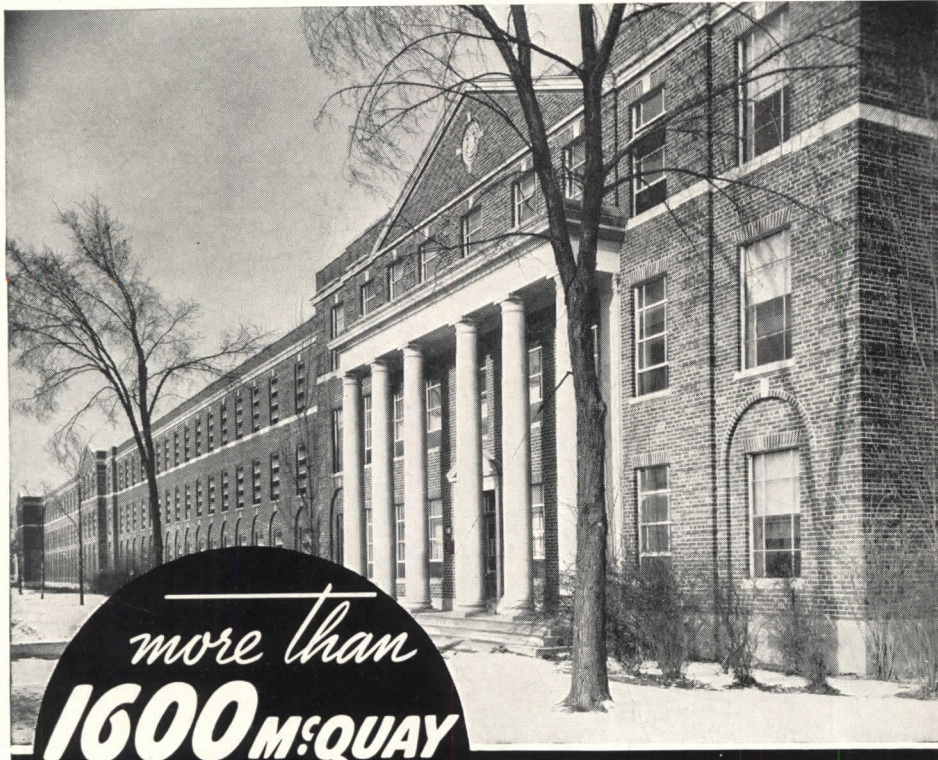
Ypsilanti State Hospital, Ypsilanti, Mich. Albert Kahn, Inc., Detroit, Architects and Engineers. Peter Eddy, Dearborn, Mich., Heating Contractor.
