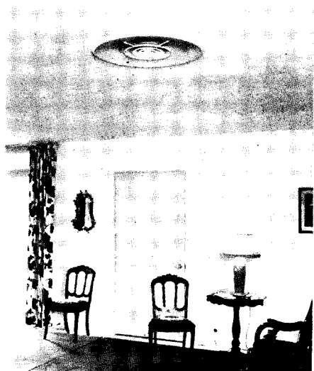
Heating and ventilating through directional air registers at ceilings
