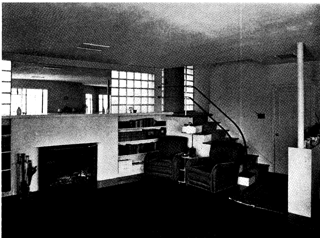
Living room on street side, 4 ft. below grade; glass block in the wall screens the room from passers-by, admitting daylight at the same time. Street door opens on a stair landing.
