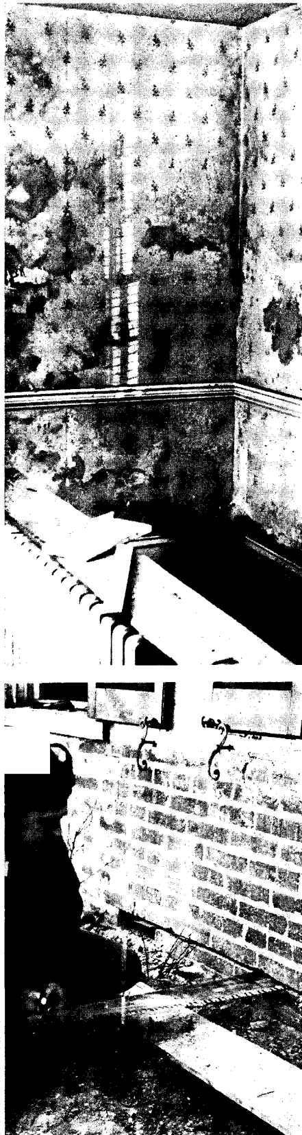
Top, damage caused by water seepage from masonry foundations. Below, preparing to install membrane waterproof by sawing wall at a brick joint
