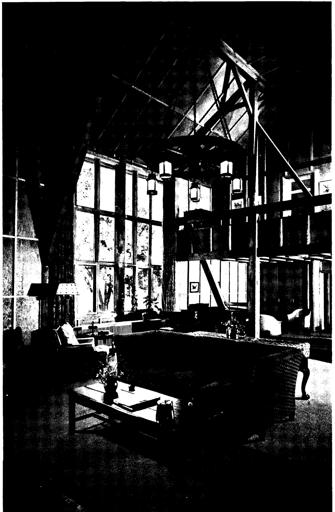
View of living room, facing north. This room is three stories high, with a balcony over one end of it. Beyond, on the balcony level, are six bedrooms and a sitting room. The walls of the living room are fir plywood; finish is natural stain. Sash are stock, cut to required size.
