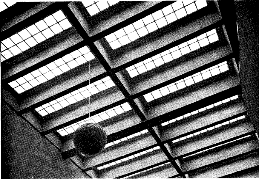
Detail of ceiling skylight. The reinforced members were poured in place. Sash are steel; glass is opaque for diffused light.
