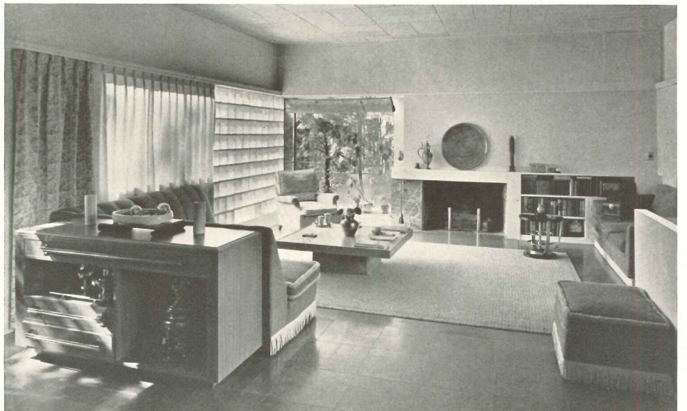
Glass block and plate glass in alternate panels vary the light transmission for living area
