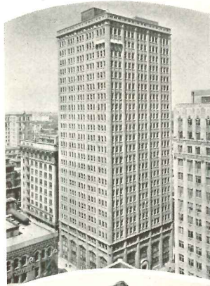
Fort Worth National Bank Bldg., Ft. Worth, Texas. Weil & Moses, consulting engineers, New Orleans. C. Wallace Plbg. Company, air conditioning, Dallas.
