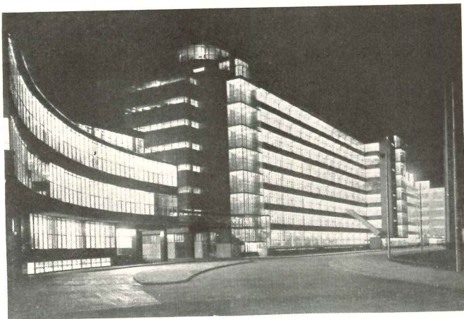
Fig. 3: AT NIGHT THE RIBBON WINDOWS do not light the factory, but the street. Looks fine, but a tremendous amount of light is wasted.
