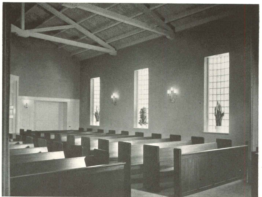
WALLS OF THE CHAPEL are painted a cool green; trim is white. The ceiling is of thick structural insulating slabs which span the purlins.
