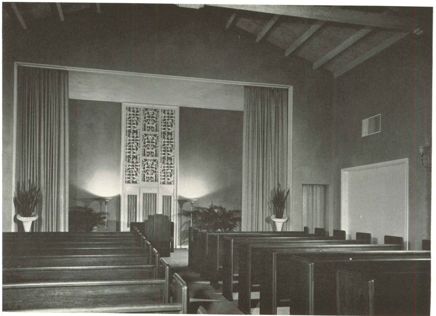
WALLS OF THE CHAPEL are painted a cool green; trim is white. The ceiling is of thick structural insulating slabs which span the purlins.
