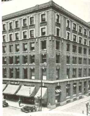
Georgia Power Company Building, Atlanta, Georgia. Air conditioning by the Atlanta Office of York Ice Machinery Corporation, York, Pa.
