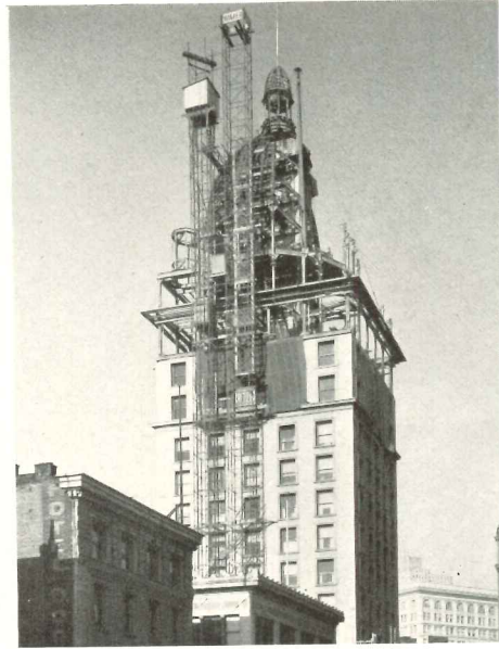
PROGRESS SHOTS show most spectacular part of the job of remodeling San Francisco's historic Claus Spreckels Building (later the Call Building) into the new Central Tower. Left, the original, which withstood the 1906 earthquake, as it was April 15. September 15: hoist-cage up, preparations for removing uneconomical upper stories in progress. November 15: dome half down, cornice masonry removed . . .
