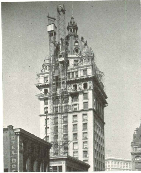
PROGRESS SHOTS show most spectacular part of the job of remodeling San Francisco's historic Claus Spreckels Building (later the Call Building) into the new Central Tower. Left, the original, which withstood the 1906 earthquake, as it was April 15. September 15: hoist-cage up, preparations for removing uneconomical upper stories in progress. November 15: dome half down, cornice masonry removed . . .
