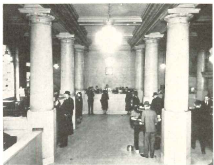
OLD (below) and NEW main banking room
