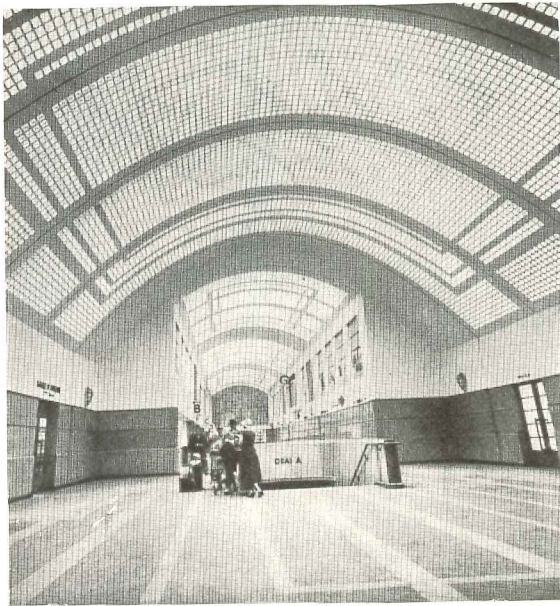
Fig. 20: GLASS-CONCRETE CONSTRUCTION, using lenses with silvered lateral surfaces, transforms the wall into a translucent screen.
