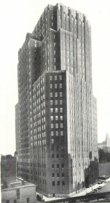
LONG DISTANCE BUILDING, NEW YORK CITY; Voorhees, Walker, Foley and Smith, Architects
