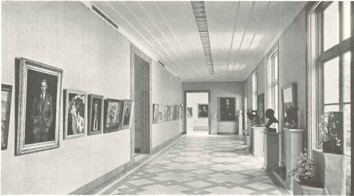
CORRIDOR GALLERY opens into patio
