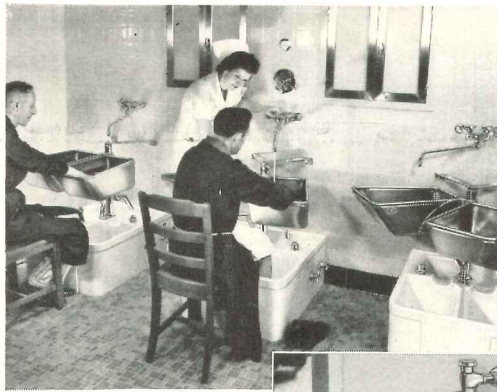
Many Crane hospital fixtures are made of Duraclay—an all-ceramic material which does not crack, craze or stain, and which is immune to thermal shocks.
