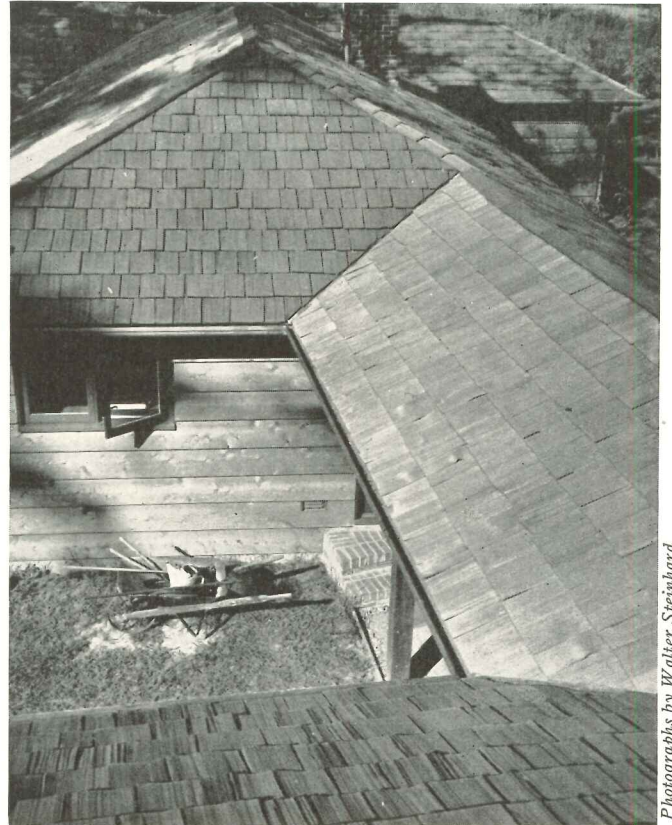
WOOD THROUGHOUT. Roof is of cedar shakes
