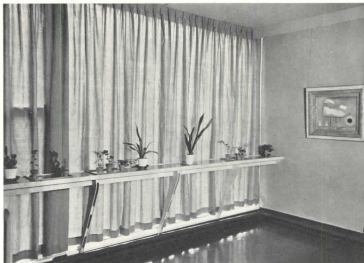
1. WEST (WINDOW) WALL. The plant shelf is supported by braces and ceiling wires, providing clearance for full-length draperies
