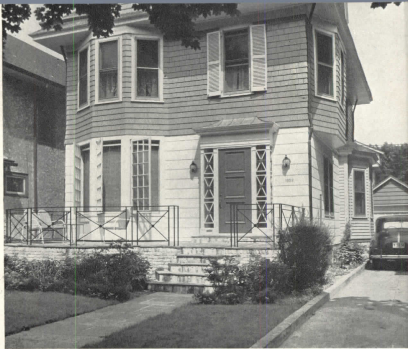
RENOVATED EXTERIOR. White composition shingles resurface the first floor; terrace of brick and slate
