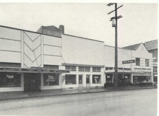
FACE LIFTING OF SIMPSON AVE., HOQUIAM, WASH. HAROLD K. WILSON, ARCHITECT. Old fronts were trued up with nailing strips. Following line production methods, exterior plywood was applied in various patterns, and fresh coats of paint completed the job—with minimum use of “short” materials. The project took 30 days; its cost was $1,200
