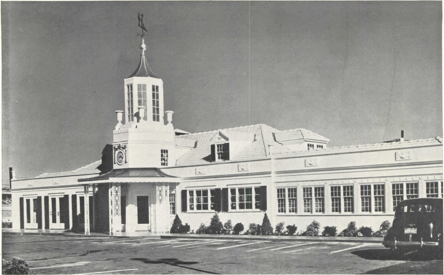
HOWARD JOHNSON RESTAURANT, CAMBRIDGE, MASS. JOSEPH MORGAN, ARCHITECT. Even this well-established chain needs its face lifted periodically, as witness this example which has recently been entirely resurfaced, on the exterior, with weather-resistant fiberboard.
