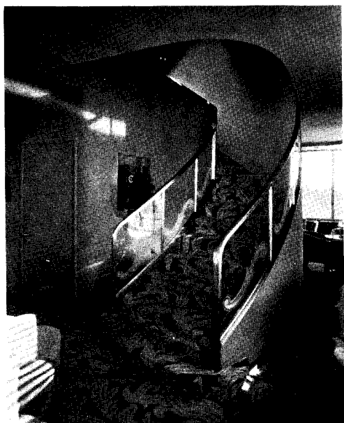
ABOVE, stairs to lounge. Rail is bronze with sand-blasted Lucite panels which house fluorescent lights. RIGHT, lounge interior. General contractor was M. H. Golden. Windows in Sky Room have heat-absorbing glass to reduce sun heat load
