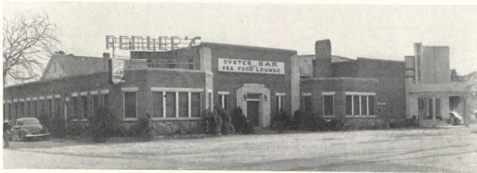
EXTERIOR of completed structure
