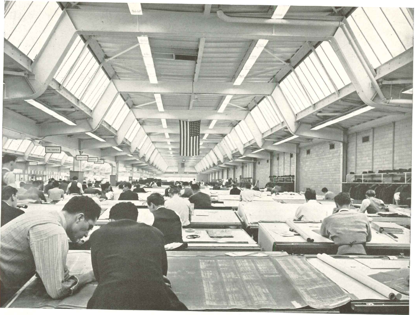
DRAFTING ROOM. Rigid frame design with bent beams provides uninterrupted light distribution from inclined monitor
