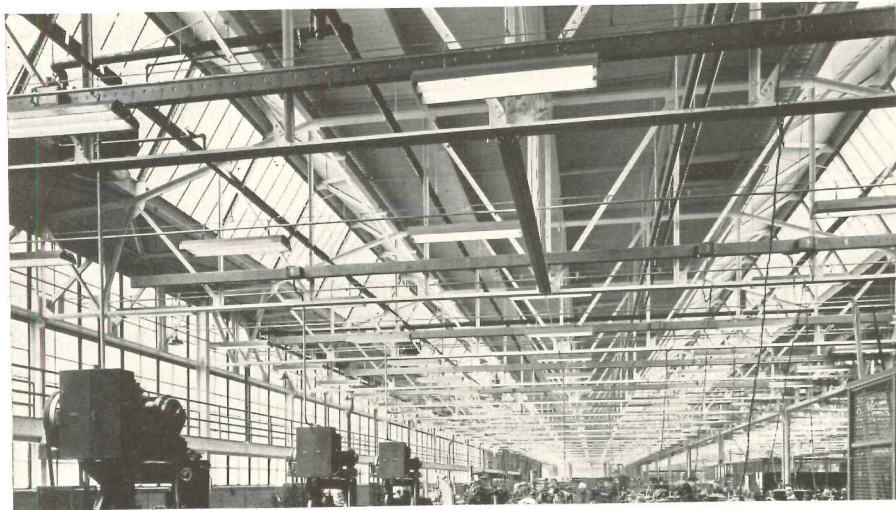
FLEXIBLE POWER DISTRIBUTION. Bus bars with outlets at 12-in. intervals allow freedom in machine placement or relocation
