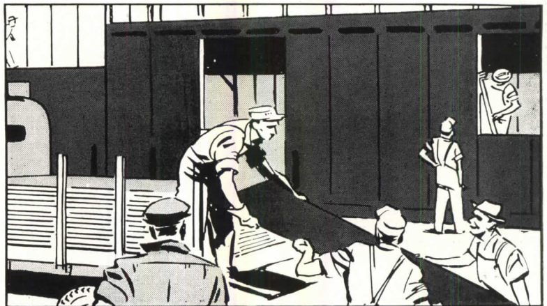
Gold Bond Exterior Board —is an extra thick gypsum board with a durable overcoat of asphalt roofing. A combination sheathing and siding which comes in large sizes covering up to 20 square feet in one operation—really saving workers' time—sturdy, rigid, permanent finish.
