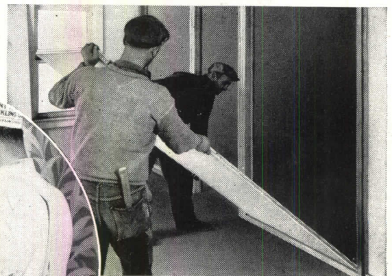
Gold Bond 1" Solid Partition Panels —save lumber—save time—build solid, rigid construction. No nails are used except to hold wooden mouldings, and panels can be completely salvaged when temporary structures are torn down.
