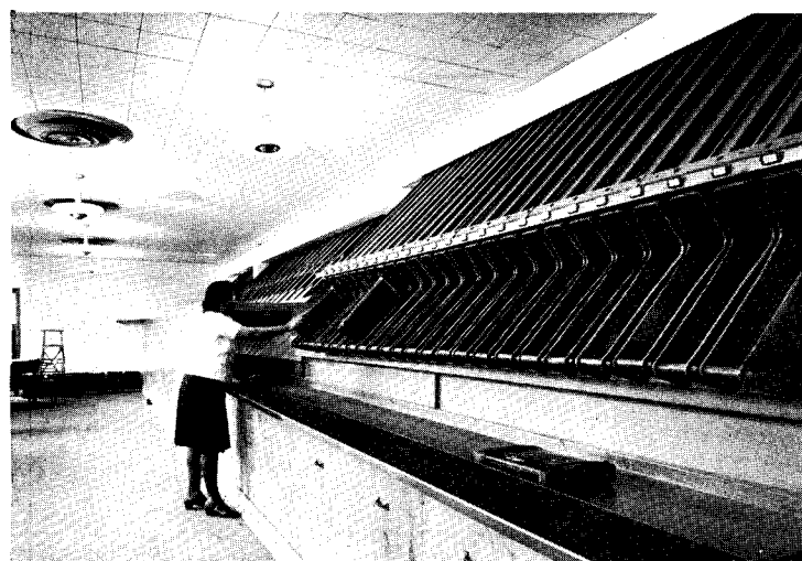
Pneumatic tubes for interoffice communication save many messenger miles
