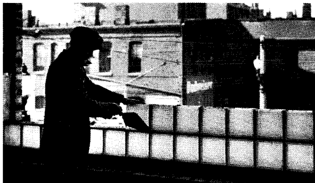
Any competent bricklayer, using regular equipment, can lay up INSULUX Glass Block panels. Little or no metal is needed for replacement panels like this one.
