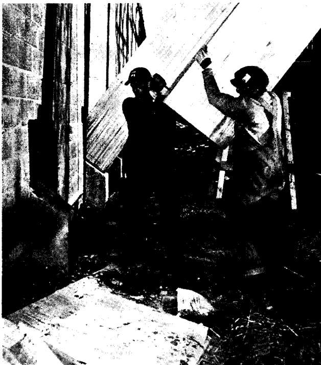
Swinging arch ends into position against concrete buttresses
