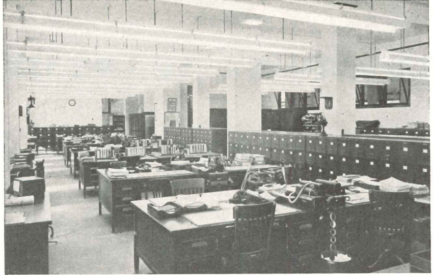
22. A good approximation of indirect lighting, from fairly inconspicuous hung fixtures which allow some of the light to leak out to illuminate the ceiling
