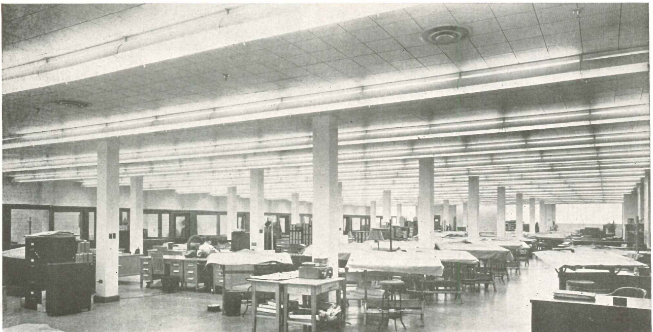
17. In this drafting room the fixtures are hung conventionally, but tables are placed diagonally, for almost shadowless lighting. (Reed Roller Bit Co., Houston)
