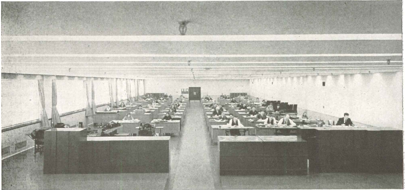
18. Fluorescent lighting in strips recessed in the ceiling gives Otis Elevator workers good seeing conditions, without the usual clutter of hung fixtures
