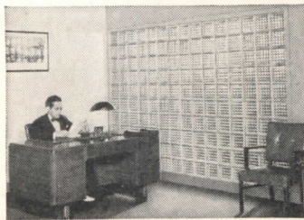
The partitions transmit daylight from office to office and provide a measure of privacy along with light.
