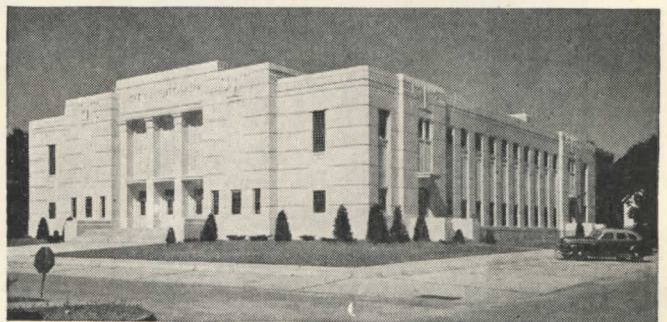
City Auditorium, York, Neb., designed by Meginnis & Schaumberg, architects, of Lincoln. Architectural concrete details produced by use of milled wood and plaster molds. Smooth exterior concrete walls cast in plywood forms.
