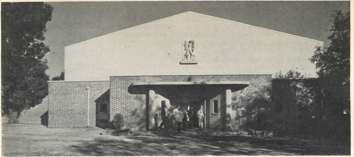
Above and below: Gymnasium of Lakeside Union School, California, Frank Wynkoop, A.I.A., Architect. A type of school room requiring special heating by unit electric heaters, as seen in the interior view
