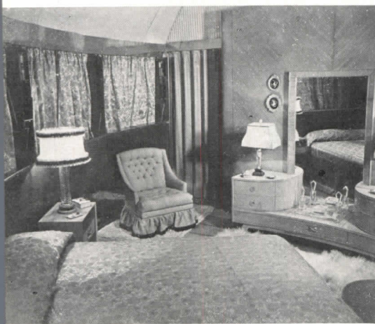
Photographs taken in the Fuller House erected at Wichita show why housewives are enchanted. Note domed ceiling, continuous drapery valance, plastic-covered accordion doors. Below, sections show switch-operated "ovolving" shelves, compact bath units, and wall with plastic curtain raised to expose plastic-screened ventilating strip below windows
