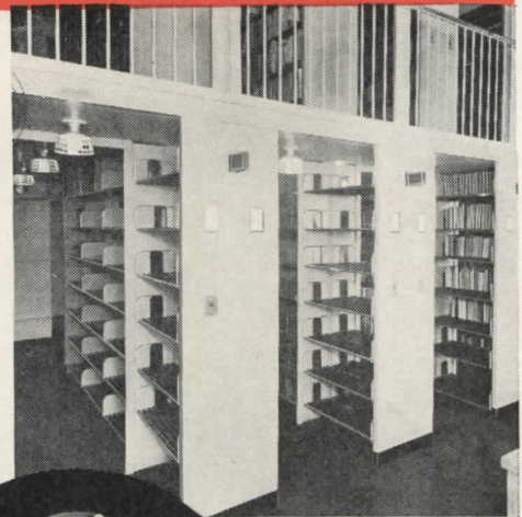
Snead Bracket Stack with heavy steel columns supporting concrete deck floor. Gallery fascia topped with Snead Railing. Stack illuminated with Snead Reflectors specially designed for the peculiar and exacting requirements of adequately illuminating the narrow aisles between book ranges.
