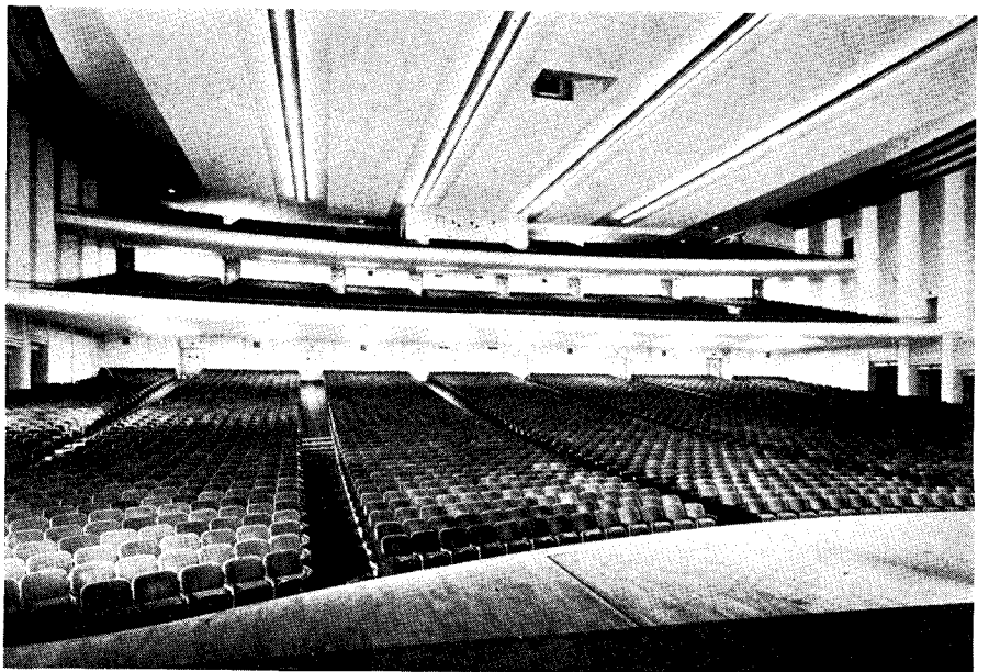
Fig. 11 and 12: Two views of Purdue University Music Hall, Walter Scholer, architect. Reflections broken by balconies, paneled rear wall surfaces, and sound-absorbing materials
