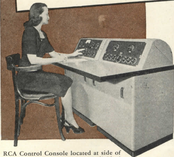
RCA Control Console located at side of balcony provides simultaneous, individual control of twelve stage microphones and auditorium volume level.
