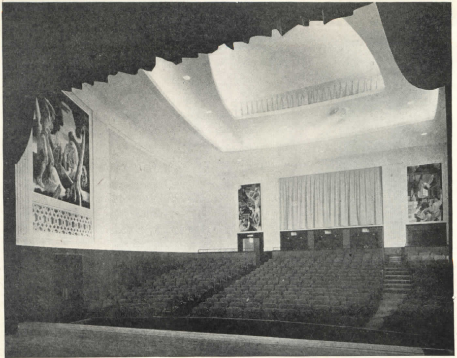
Fig. 15: Indiana University Theater. Walls funnel in toward the stage, walls and ceiling being paneled with sound-absorbing material and broken surfaces to control sound
