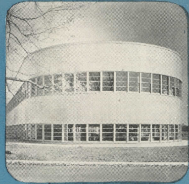
Faced entirely of Alcoa Aluminum sheet this building is tangible evidence of the trend to aluminum for building construction.
