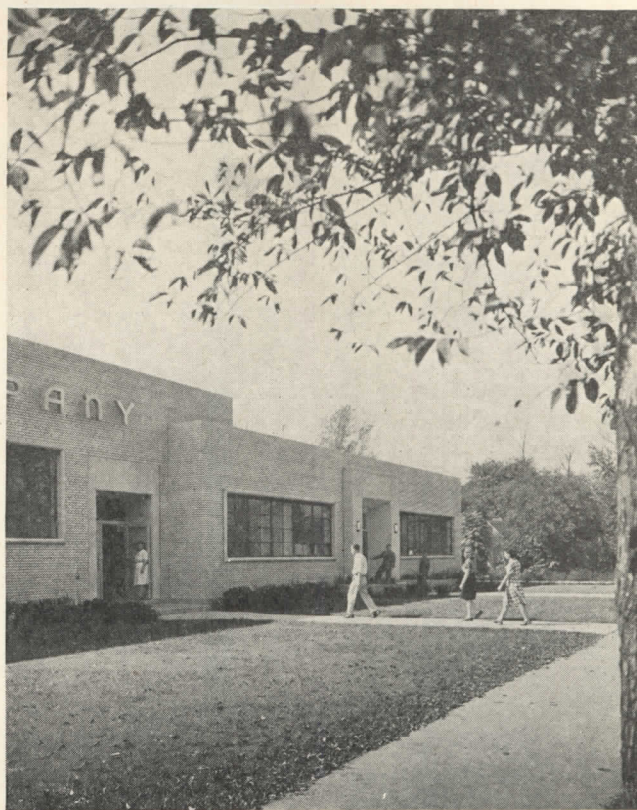
Right: it was not by accident that the employee entrances were placed at the front. Office portion in the background has its own entrance. Below: the orderly row of printing presses, with the wide aisle for skid-truck paper handling, is a good illustration of the advantages of the wide column spacing in the modern plant
