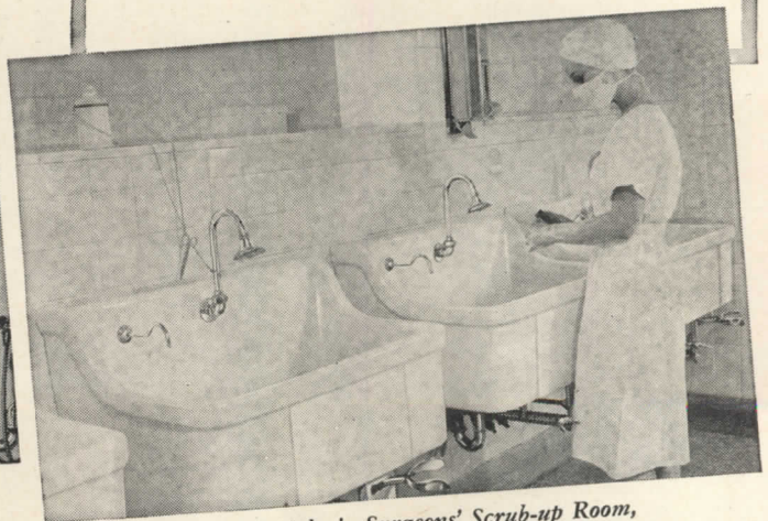
Duraclay sinks in Surgeons' Scrub-up Room, St. Francis Hospital, Evanston.
