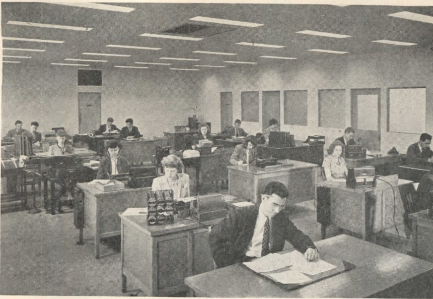
Sound-treated ceiling and recessed fluorescent lighting of 35 footcandles, plus air conditioning, make for comfortable working conditions in the office portion. Sprinkler pipes are concealed in ceiling
