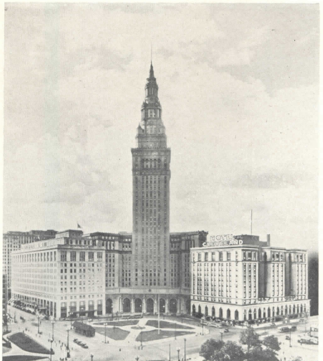
HOTEL CLEVELAND CLEVELAND, O. Small, Smith & Reeb, Architects
