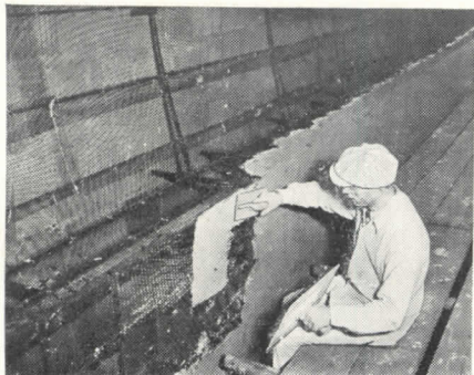
CORROSION RESISTANT! Wet plaster . . . between-wall condensation . . . lime-bearing seepage never get far against Monel. This rustproof Nickel Alloy resists corrosion by alkalis and salts in plaster, lime and other building materials.
