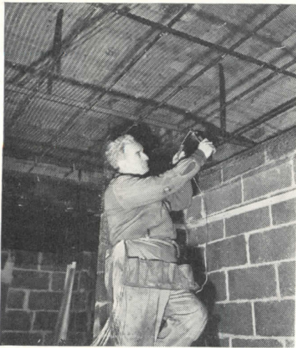
DUCTILE! Monel* tie-wire is pliable . . . easy-handling. And it's solid metal . . . corrosion-resistant all the way through . Has no coating that flakes off when the metal lather bends it. Twists to a snug fit without breaking!
