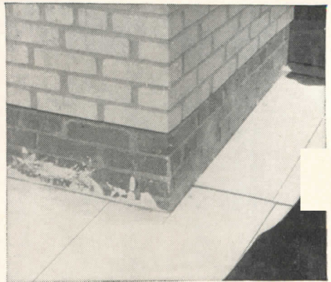
EASY TO FIT. Kaylo Insulating Roof Tile can be cut and fitted with ordinary hand or power tools. Picture above shows example of re-entrant cut made to fit around stack.
