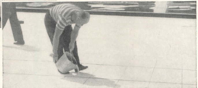
EASY TO FIT. Kaylo Insulating Roof Tile can be cut and fitted with ordinary hand or power tools. Picture above shows example of re-entrant cut made to fit around stack.
