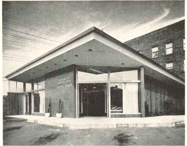
University National Bank Parking Lot Branch, Seattle, Wash., Smith, Carroll & Johanson, archts.: designed for inside service
