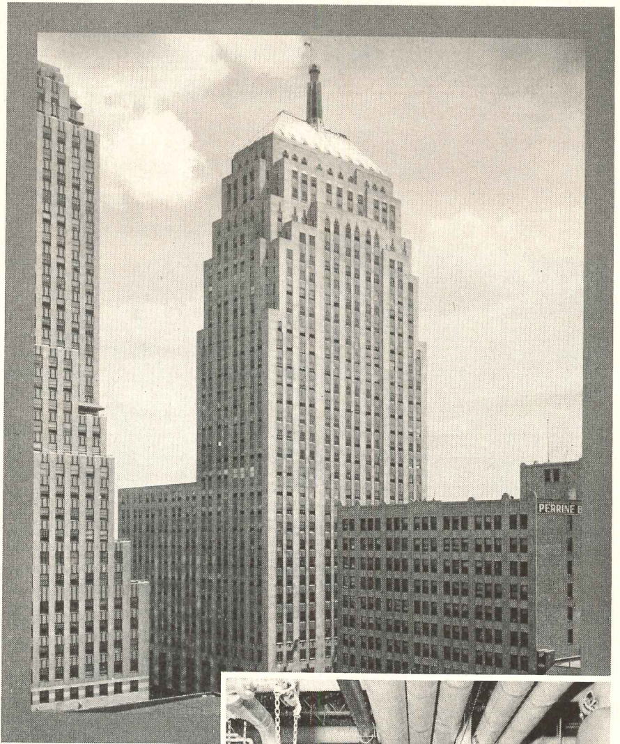
First National Bank Building, Oklahoma City, Oklahoma. Sorey, Hill and Sorey and Ira G. Howlett, Architects. Spaeth Engineering Company, Piping Contractors.
