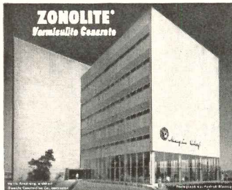
Above: The ultramodern American Stove Company in St. Louis has a monolithically poured Zonolite concrete roof... specified by Harris Armstrong, architect, for its lightness, strength and fire protection.
