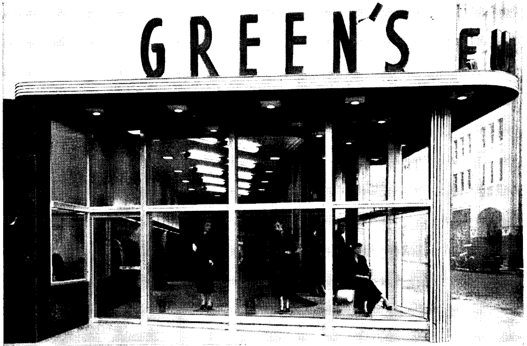
Architects: Erhart, Eichenbaum and Rauch, Little Rock, Ark. Associate Archt. L. C. Cavitt, Fort Worth, Tex.
