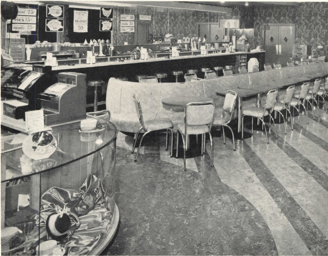
1. This beautiful floor installation in the Colonial House Candy Shop, East Orange, New Jersey, shows
