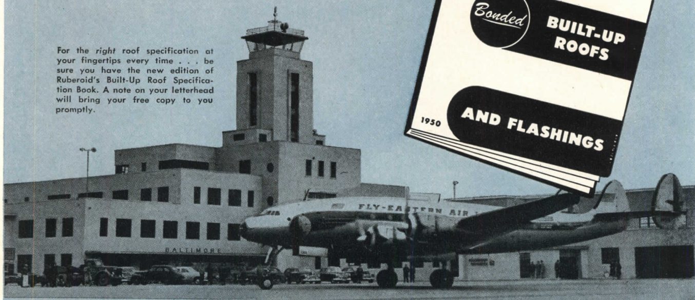
Terminal Building, Friendship International Airport. Architect: Whitman-Requardt-Greiner Co. & Asso. General Contractor: Consolidated Engineering Co. Roofing Contractor: Lloyd E. Mitchell, Inc.
