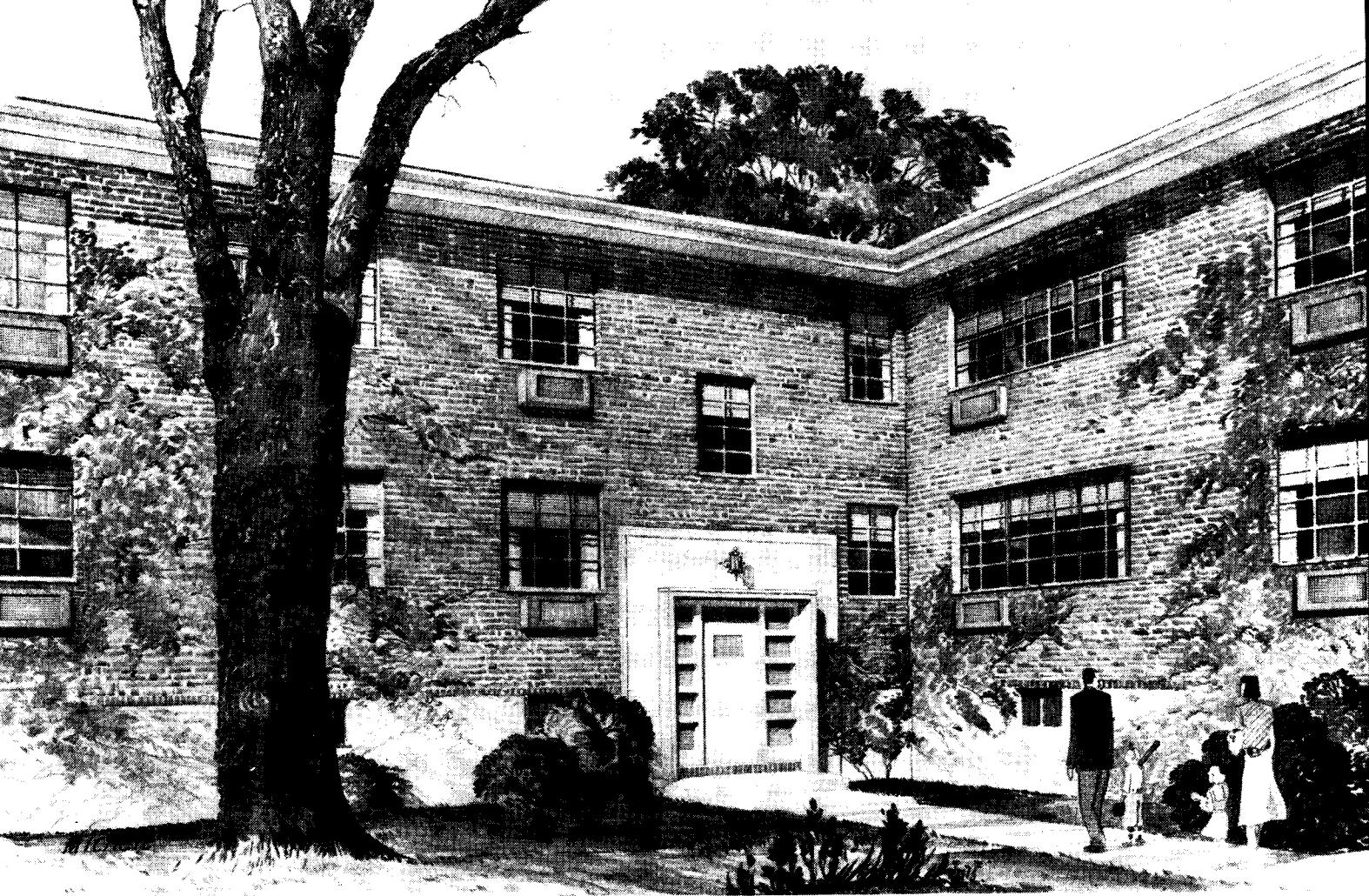
Above: Exterior of Childs Garden Apartments, showing placement of Frigidaire window air conditioners. "It is my conviction," says Robert Metrick, the builder, "that air conditioning is the greatest drawing card in attracting and holding tenants today."
