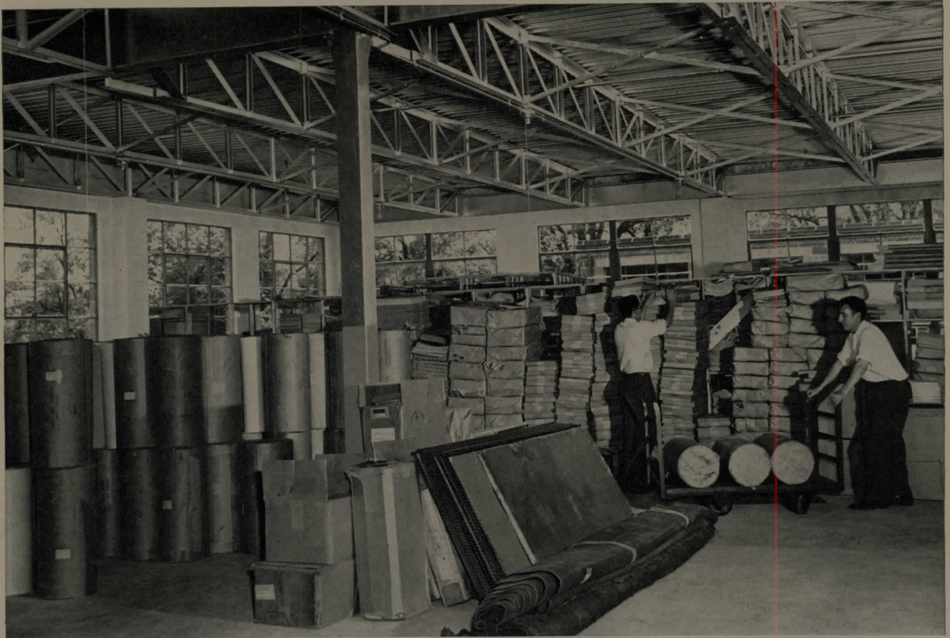
Bethlehem Longspan Joists installed in Katzenbach & Warren, Inc., warehouse, New Canaan, Conn.; Architect and Engineer: William A. Grey, Redding, Conn. Contractor: John Zandonella, Bridgeport, Conn.
