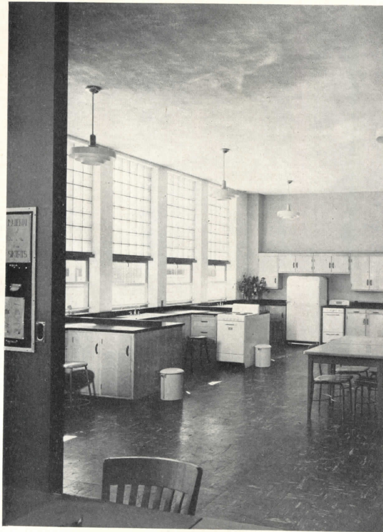
Above is home economics laboratory, with gas and electric equipment because both are in local use. Bottom right, home economics classroom, separated from laboratory by a sliding wall. Upper right, stair from lobby to second floor
