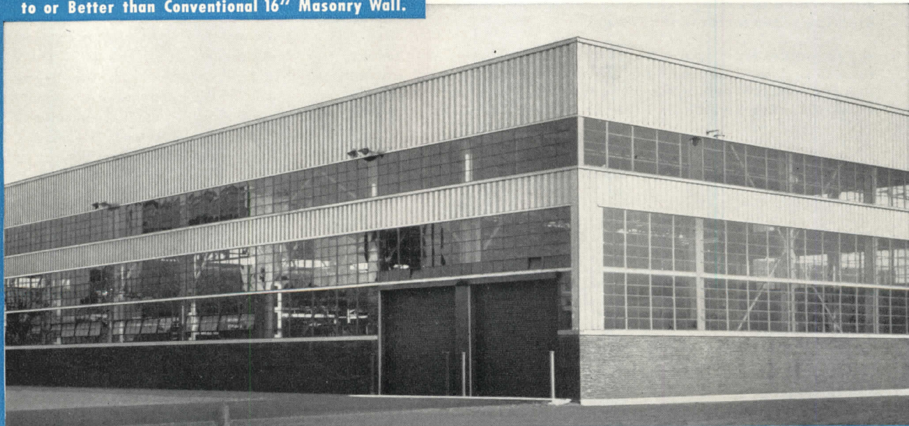
New Plant for Budd Mfg. Co. Insulated Metal Walls employed here are Mahon Field Constructed Fluted Type, with Exterior Wall Plates of Aluminum. Giffels & Vallet, Inc., L. Rossetti Archt. and Eng., S. N. Nielsen Co. Gen. Contrs.
