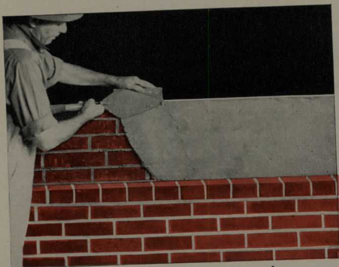
The face brick should be backplastered.
