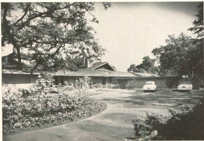
Residence of stone and redwood for Mr. and Mrs. Arthur Hanisch, Pasadena. Architect: Henry Eggers; assoc., Walter Wilkman
