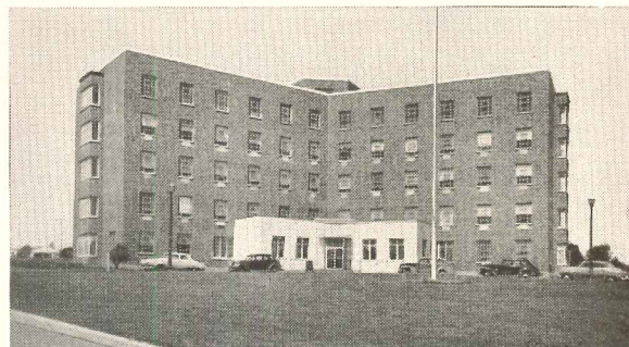
Frigidaire Air Conditioning and Refrigeration throughout.
