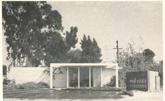
Residence and office for Mr. and Mrs. John E. Baird. Cost: $6800 for 742 sq ft, including blacktop, paving of brick, curbs, fill planting and draperies. Architect: Edward Killingsworth
