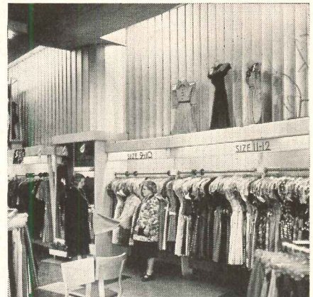
KAISER ALUMINUM SIDING , installed vertically in The Cotton Shop , Chicago, gives effect of height, fits curved surface, hides heavy columns. Baked-on enamel coat is smooth, easy to clean, lasts longer. Architects: Walter H. Sobel, J. Stewart Stein. Contractor: Lee Construction Co., Chicago.
