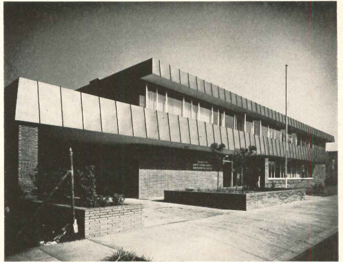
Administration Building, Culver City Unified School District, Culver City, Cal. Exterior walls are brick and copper. Architects and engineers: Daniel, Mann, Johnson and Mendenhall
