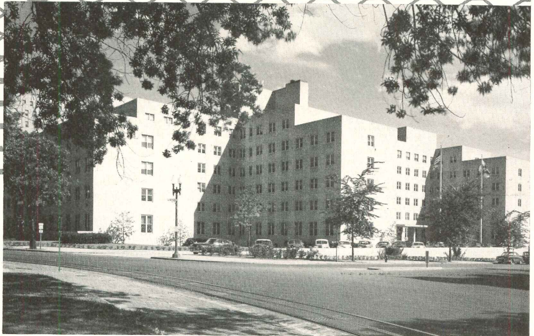
George Washington University's new hospital. Faulkner, Kingsbury and Stenhouse, Architects. Charles H. Tomkins Company, General Contractors.
