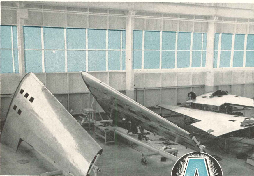
SIDEWALL INSTALLATION at Douglas Aircraft Plant, El Segundo, Calif.—corrugated metal siding was removed and replaced with Alsynite panels. No additional framing required. Lap-joints sealed with mastic. Light diffusion throughout interior greatly increased due to refractive action of Alsynite.
