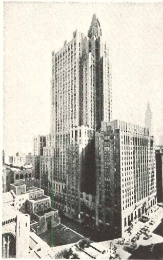
The Waldorf-Astoria in New York . . . famed for comfort and hospitality... makes extensive use of modern air conditioning.
