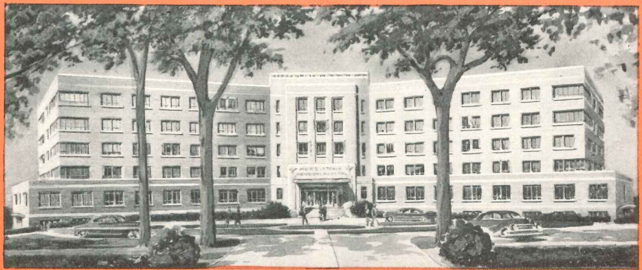
Morristown Memorial Hospital, Morristown, N. J. Architects: John H. & Wilson C. Ely, Newark, N. J. Hospital Consultant: Gerhard Hartman, Ph. D., New York City Mechanical Engineers: Meyer, Strong & Jones, New York City Contractor: August Arace & Sons, Inc., Elizabeth, N. J.
