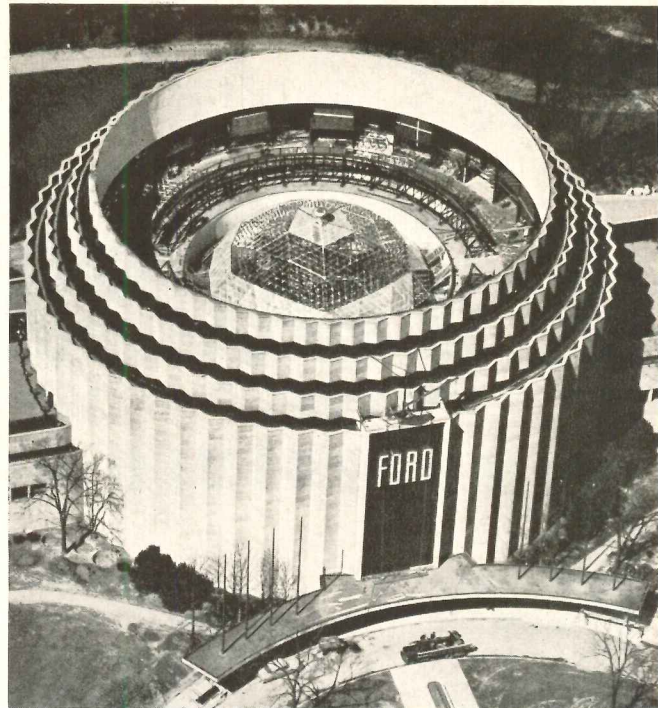
Truss being positioned on scaffolding mast (left); mast was jacked up as trusses were added
