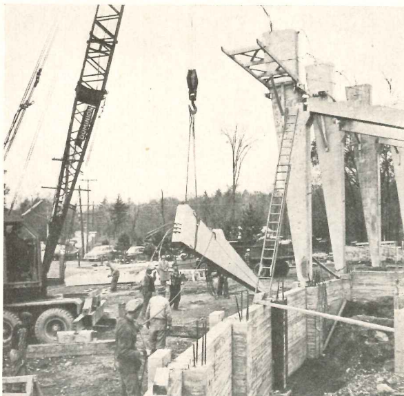
Tapered column, with unstressed cables projecting
