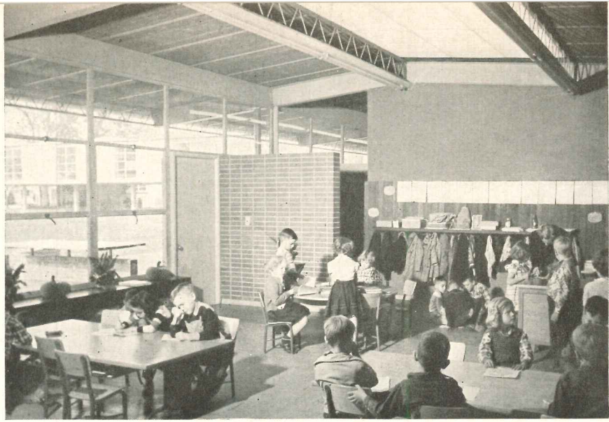
Classrooms in Sweeny school, top and bottom of page, are similar in high and low wings (low wing rooms shown). Skylighting is even, diffused, baffled by fixed Venetian blind slats. Continuous fluorescent tubes are fastened to exposed bar joists
