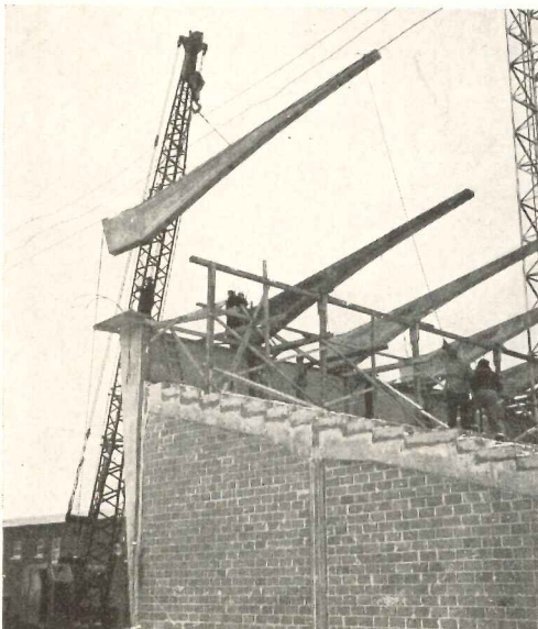
Cantilevered roof beam being lowered into place
