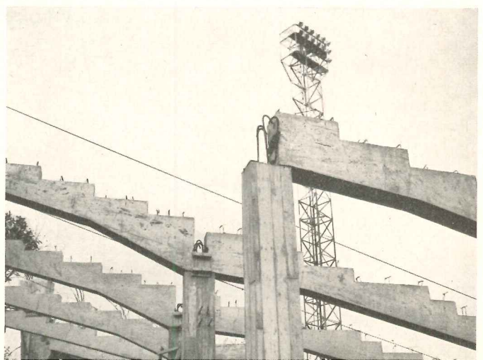
Bleachers beams resting on intermediate column; end above
