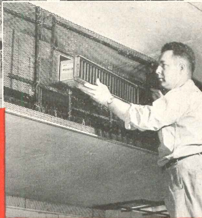
(Above) Ductwork before installation of partitions or metal lath ceilings. Complete job required 340 Air Valves, 12 High Velocity Control Units, 207 Sidewall Diffusers and Return Grilles, 10 Air-turns. (Right) Air Valve and Diffuser go into place. Valve is adjusted quickly and easily with key through face of Uni-Flo Double Deflection Sidewall Diffuser.
