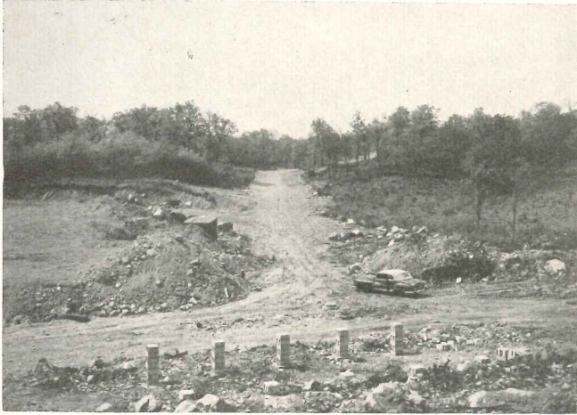
An attractive site was difficult for construction . . .
