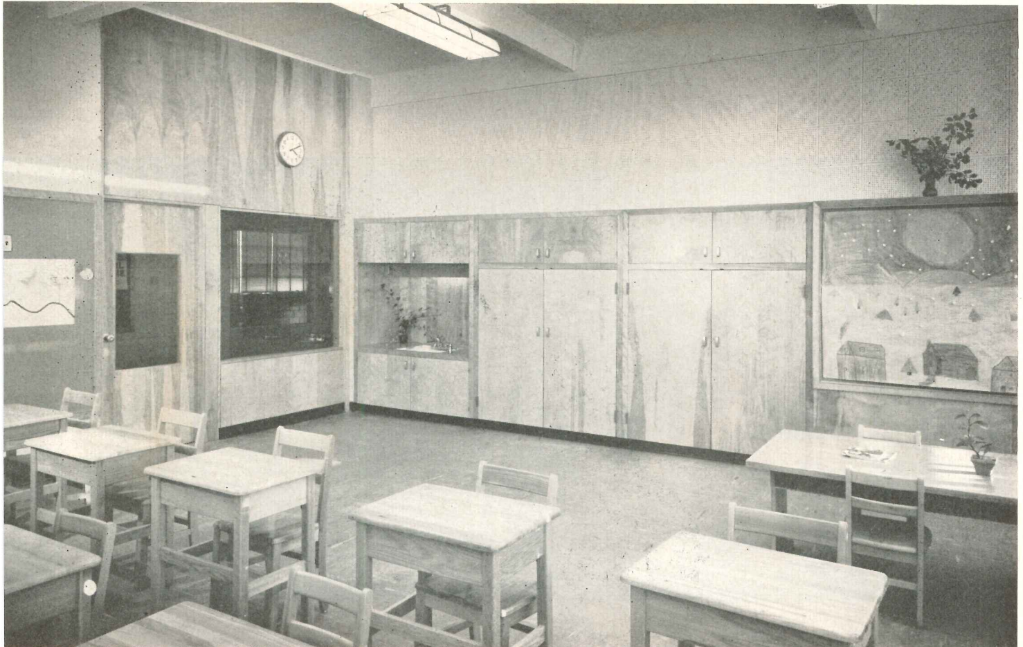
Photos of typical classroom, above and below, and drawings, left, of assembled storage partition, show backs of units supporting chalk boards and tack space for adjoining rooms. Corridor wall has large wire-glazed sash which help light — and relieve monotony of — corridor
