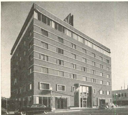
The Frederick Martin Hotel is built of brick veneer over reinforced concrete. Bethlehem supplied the reinforcing steel for the entire building.
