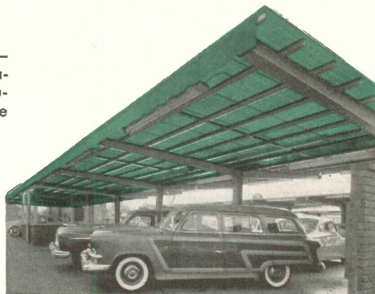
CHEM-O-GLAS UPS SALES — Outdoor showroom of J. A. Eisele Sales, Inc., one of west coast's largest Lincoln-Mercury dealers, showing utilization of CHEM-O-GLAS ribbed structural panels as roofing for structural steel carports.
