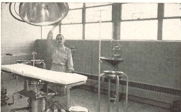
Operating Room. Webster Walvector offsets heat loss from large glass exposures here and in nursery and obstetric suite.
