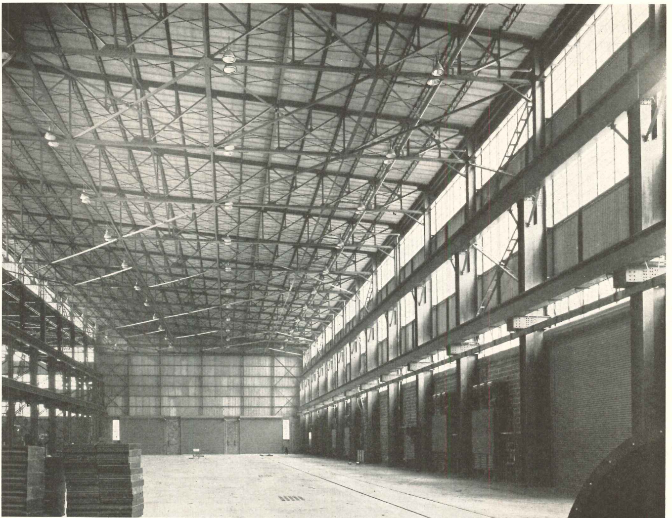
Six trunk lines under the floor of the building house utilities and air exhaust system. Branch lines connect with floor outlets (visible in photo below). Wall mounted unit heaters supply air in winter. Large blower fans outside building (across page) pull air through exhaust system
