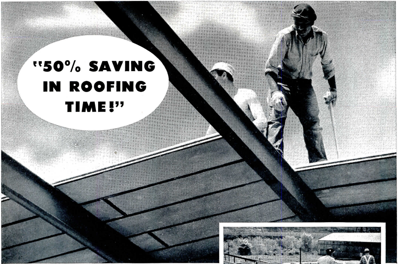
C & D Batteries, Inc., plant at Conshohocken, Pa. Building Contractors: Lloyd F. Kershner, Inc., Norristown, Pa.
