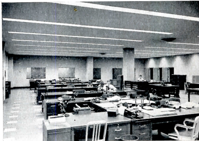
THE EVENING SUN'S EDITORIAL ROOM. Quiet now, but full of active, fast-working people before press time. And the light they work by helps them get the job done right, never hinders them. The fixtures are Day-Brite's Alzak parabolic troffers. The parabolic design and diffuse Alzak aluminum provide accurate control of light distribution and an excellent low-brightness ratio.
