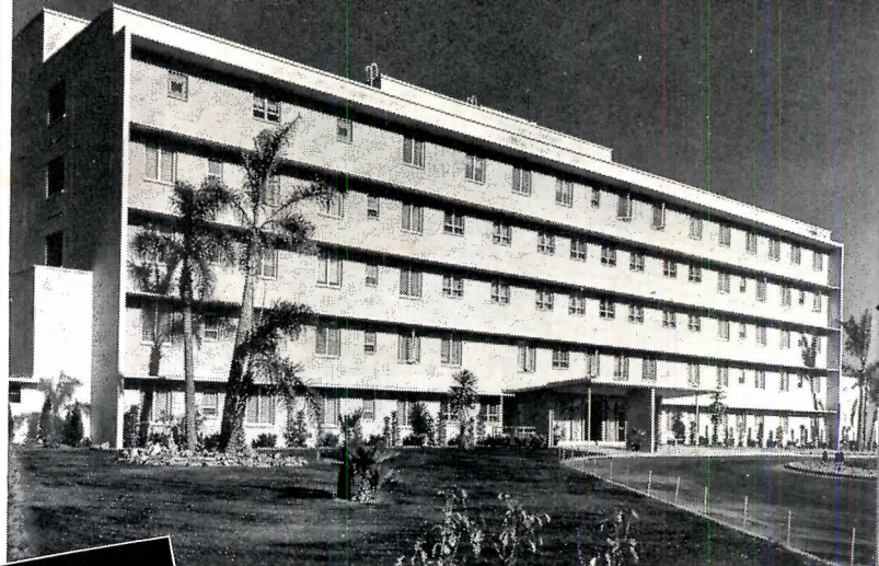
St. Joseph's Hospital Addition, Burbank, Calif. Archt.—John W. Maloney, Seattle, Wash.; Contr.—Pozzo Construction Co., Los Angeles. Pozzolith Ready-Mixed Concrete supplied by Jewel City Ready-Mix Co., Beverly Hills.
