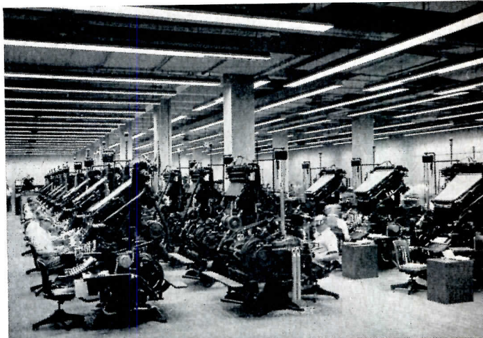
THE SUN'S COMPOSING ROOM. Even without the acoustical ceiling which is still to be installed, the Day-Brite Alzak parabolic troffers here transform this room into an extra comfortable working area, comparable to the finest office space. A sensible approach, too, because mistakes and inaccuracies are just as costly here as in the office.
