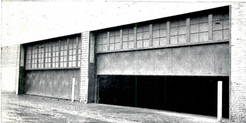
Harley, Ellington & Day, Inc. Architects, Detroit, Michigan
