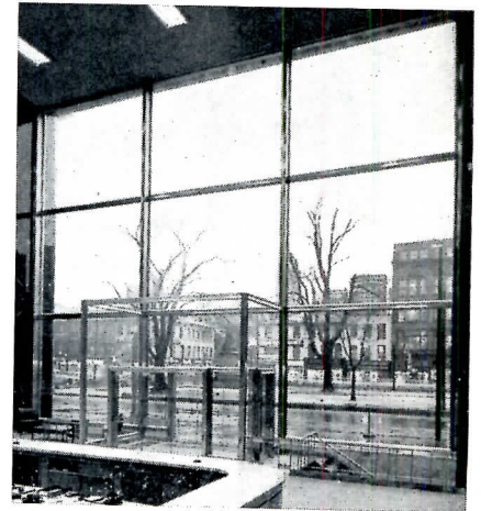
Dominant feature of the newly built Hamilton, Ont., Branch of the Bank of Nova Scotia is the plate glass window which measures 42 by 36 ft. Panes are supported by structural steel which is covered with stainless steel. Designers of the bank were McDonnell & Lenz, Hamilton architects
