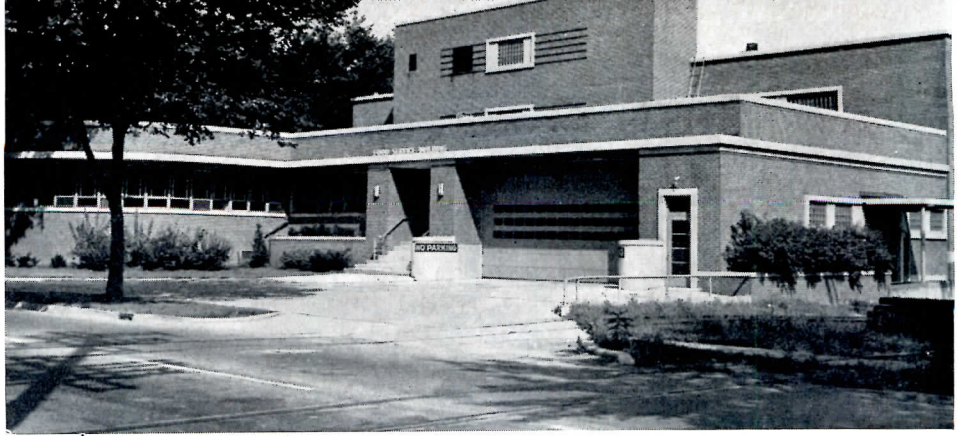
Food Service Building, University of Michigan — Louis C. Kingscott & Associates, Architects; Lynn W. Fry, Supervising Architect. Rails lead to loading dock, far right. Overhead door raises to admit trucks
