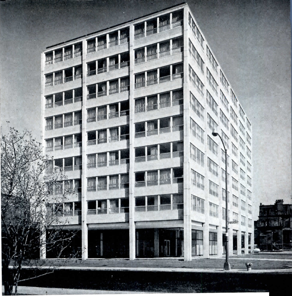
Carman Hall, recently completed student-staff apartment building
