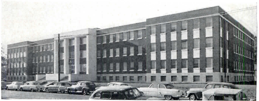
Men's dormitory for Baylor University (Texas) accommodates 340, cost $700,000. Area per occupant, 176 sq ft; study-bedroom, 107 sq ft; toilet-shower, 10 sq ft. Architects: Easterwood & Easterwood
