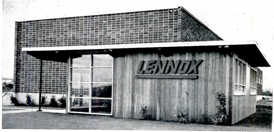
Recently completed in Calgary, Alta.: a new office and warehouse for the Lennox Furnace Co. (Canada) Ltd., designed by architects Rule, Wynn & Rule of Calgary and Edmonton
