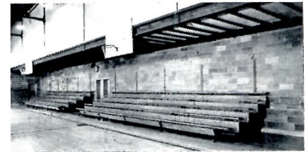
Long Island Jack Knife Bleachers, supported by steel bearing plates, fold away. Long Island Bleacher Co., Inc., 33-35 Ninth St., Long Island City 6, N. Y.
