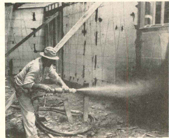
Styrofoam walls were prestressed by wires strung from ceiling to floor, then were strengthened with 1 in. of sprayed cement on both sides. On some floors marble slices were bonded to Styrofoam
