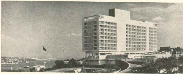
Istanbul Hilton Hotel, Turkey — Owner, Turkish Republic Pension Fund; Architect, Skidmore, Owings & Merrill, Sedad H. Elden; Structural Engineer, Prof. Said Kuran; Interior Design, Jane Kidder, Director; General Contractor, Julius Begger, Dyckerhoff Widman (AR, January 1953, pages 103-116)
