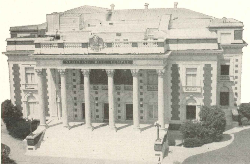
Masonic Temple, Dallas, Texas—The roof was coated with Karnak Aluminum-Asphalt Coating by Wright Waterproofing Co., Dallas
