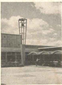
COVER: Abraham Lincoln Junior High School, Wyandotte, Mich.; Eberle M. Smith, Associates, Architects-Engineers; Lens-Art Photo
