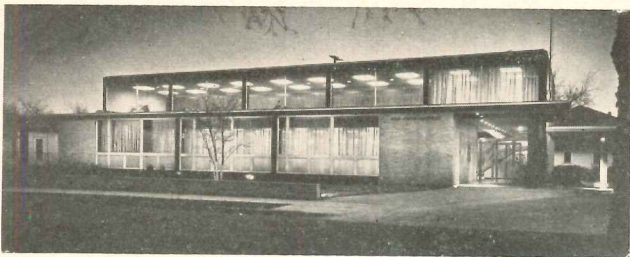
Building for Oak Cliff Savings & Loan Association, Dallas, Tex. — Architect, Prinz & Brooks, Dallas; Mechanical Engineer, Arnold Gaynor; Contractor, Burgher Construction Company
