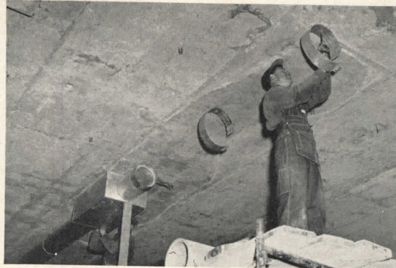
Metal gasket-strap are fastened to inserts in concrete slab
