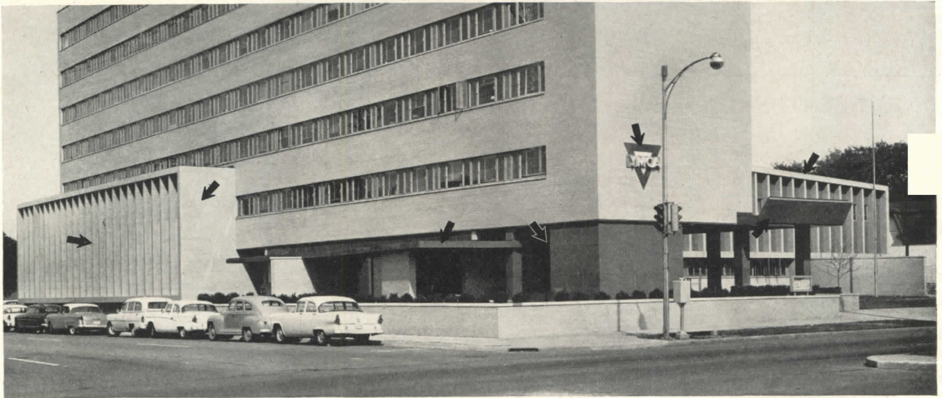
Y.M.C.A. BUILDING, PEORIA, ILLINOIS Architects: Gregg & Briggs General Contractor: Fred Harbers Sons, Inc.
