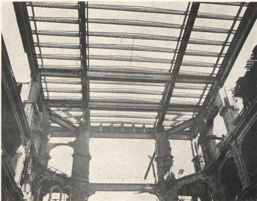
Skylight of the arcade which covered original court
