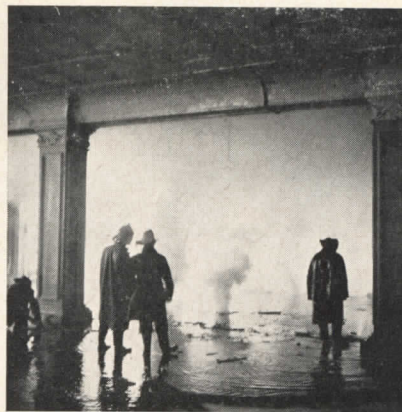
Fire started before main demolition got under way; was worst in New York for 30 years.
