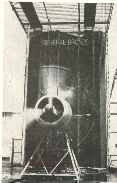
Propeller drives water from overhead pipes against building mock-up
