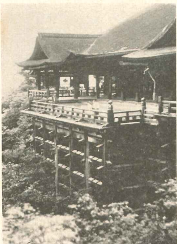
Platform supported by columns
