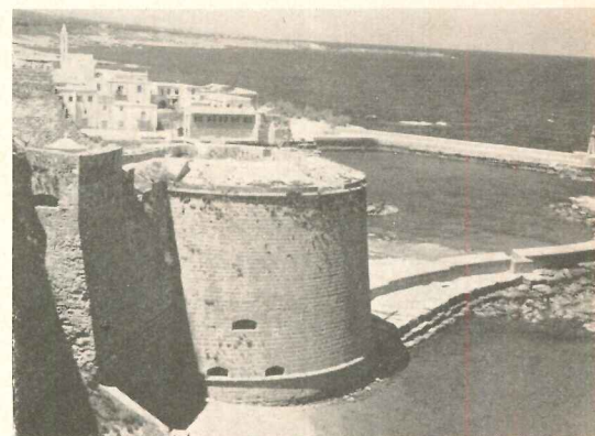
Walls adapted to the terrain
