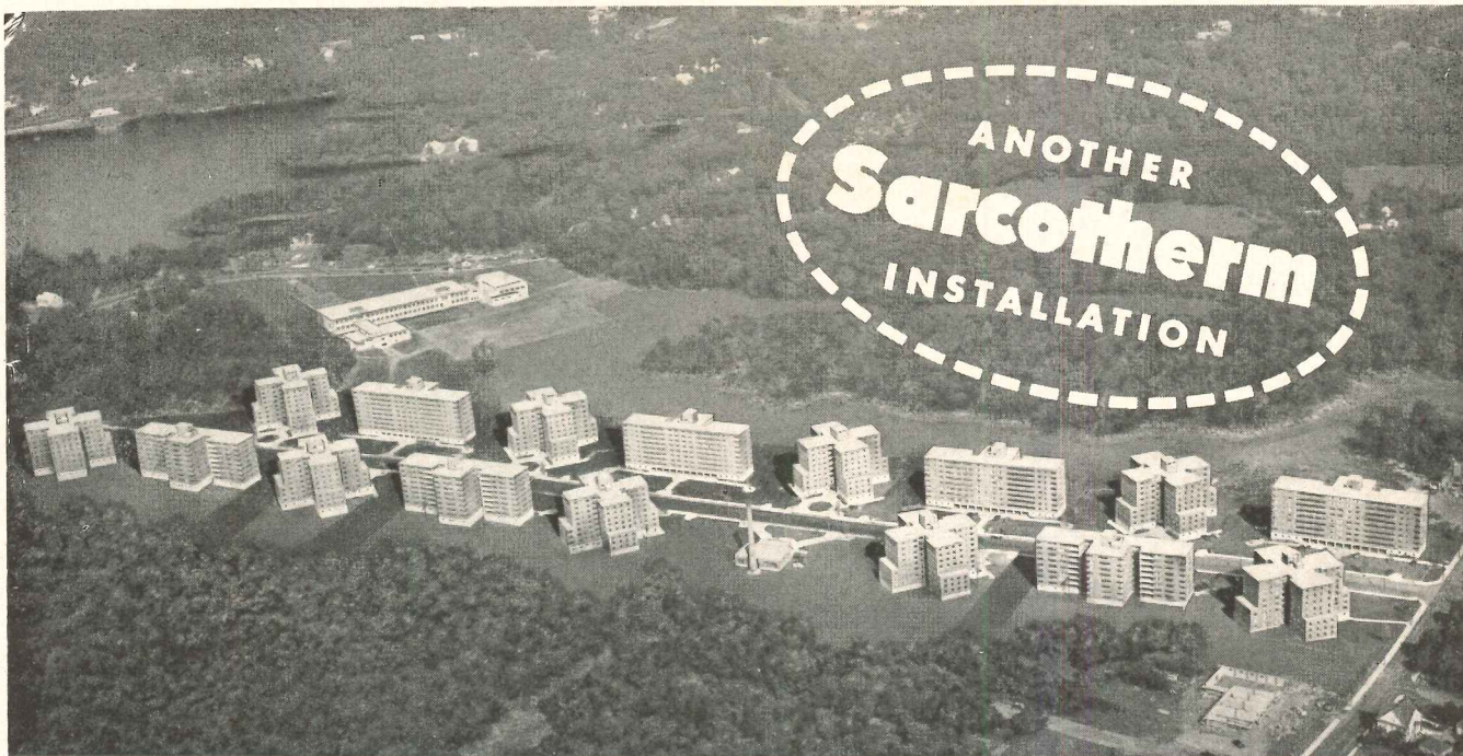
Beardsley Terrace Housing, Bridgeport, Conn. • Engineers: Frederick M. Hill and Paul D. Harrigan, New Haven. Architects: Lindsay & Johnson, Bridgeport. • Heating Contractor: Bridgeport Pipe & Engineering Co., Bridgeport. • General Contractor: E & F Construction Co., Bridgeport.
