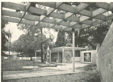
pavilion (center) is composed of six bays of 18 ft span prestressed periphery beams which carry a 3 ft grid of post-stressed
