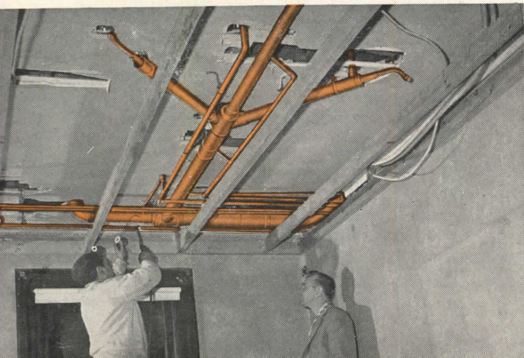
Simplify remodeling jobs. Lightweight copper tube and solder-joint fittings made light work of an otherwise back-breaking job, in adding two baths in this remodeled residence. Note how little ceiling height was lost.
