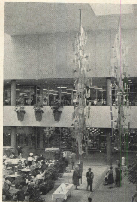
The Garden Court, 109 by 270 ft, acts as a plenum chamber to supply 70 F ventilation air to Dayton's store and tenant stores. Air enters
