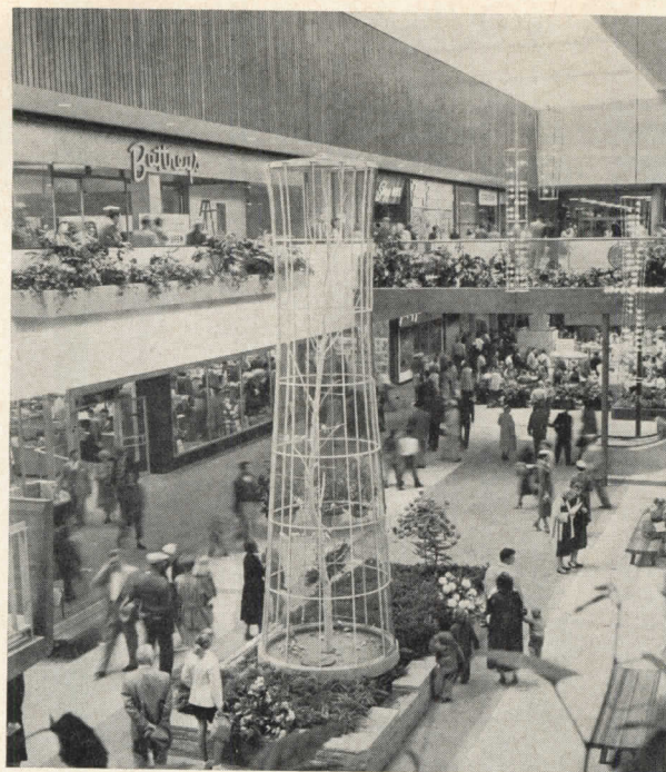
The Garden Court, 109 by 270 ft, acts as a plenum chamber to supply 70 F ventilation air to Dayton's store and tenant stores. Air enters
