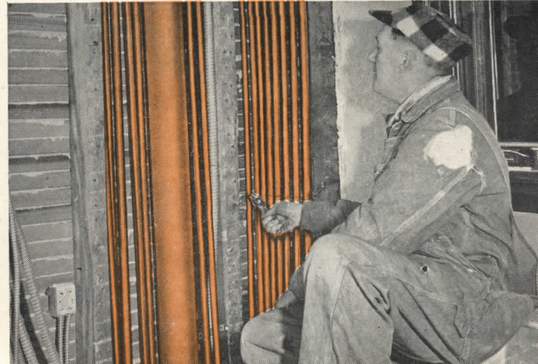
Trim, compact lines. In this remodeling job, two stud spaces served as the chase for the copper tube risers. The large tube is the soil stack; smaller tubes are water supply and heating lines.
