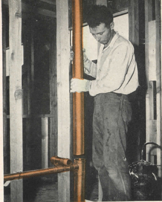
Tube and fittings fit in standard partitions. A 3" copper tube stack with fittings can be installed within a standard 4"-wide stud partition.
