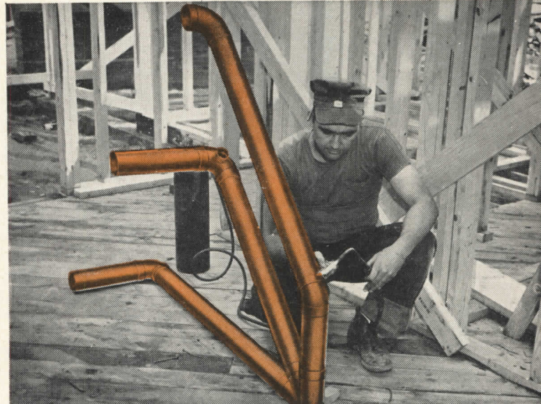
Prefabrication speeds construction. Sections like this can be preassembled out in the open or at the shop where men can work easier and faster—no lost time waiting for construction.
