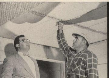
Eby (left) inspects application of Keycorner, used to reinforce joints. Keycorner is also used at all wall and corner junctures.
