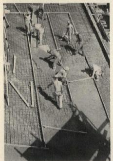
Wire-reinforced shell is poured in place
