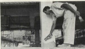
Applying fireproof Zonolite vermiculite plaster to columns.
