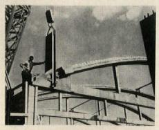
Vertical hanger posts made up of groutfilled 8 by 8 in. units and mild steel bars support bottom chord. Roof is of 6 in. pretensioned soffit block planks
