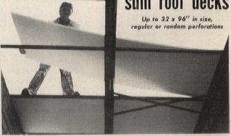
Only Hansotone\* Perforated Acoustical Formboard offers the size and strength, speedy installation and rigid permanence that add up to such LOW COST per square foot. Its outstanding acoustical qualities and high thermal insulation assure a truly efficient, attractive base for economical poured-in-place gypsum roof decks. Its white factory shop coating with .76 light reflection makes up easily into acoustical ceilings and even walls at no extra cost for finishing.
