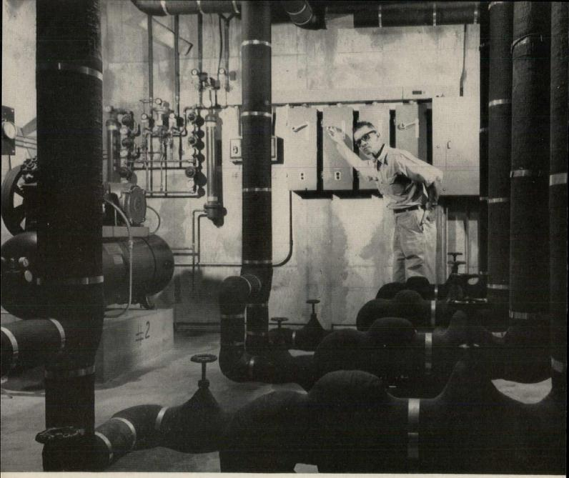
Illustration shows the utilization of individual Westinghouse motor controls. The four vacuum pumps in the foreground are individually controlled by the motor controls being operated in the background.
