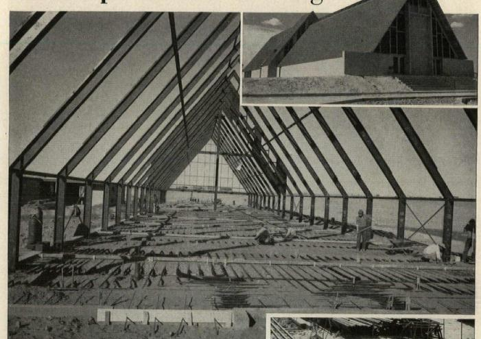
Steel Pipe Radiant Panels in main auditorium, 1" standard black pipe on 12" centers.
