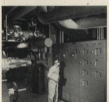
One of the two motor control centers with Type B wiring installed in hospital by Westinghouse. Each starter has 480-to 110-volt individual control transformer.
