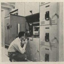
OPERATING EASE, reliability of G-E drawout switchgear with AK-1 breakers provide safer switching of 480-v feeders.
