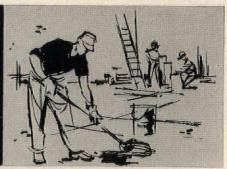
Roofing felt is mopped into position. Built up roofing completes the deck and ceiling construction. Three operations and the job's completed.
