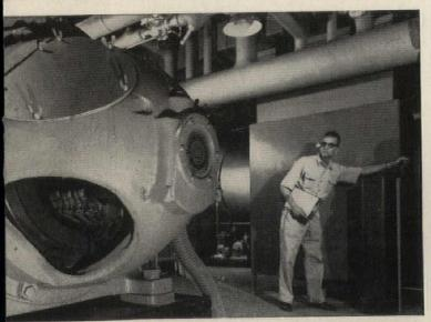
Operator is adjusting rpm of one of two 250-hp compressor motors. On-off switch is on column at right and motor control components are in large enclosed cabinet.
