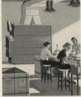
For an engineering-drafting room, quiet Carrier Weathermakers can discharge draft-free air without any ductwork. The Multi-Weathermaker System permits air conditioning in one area while the System is shut off elsewhere.
