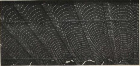
Underside of forms can be left exposed as above, painted, or used to support hung ceiling
