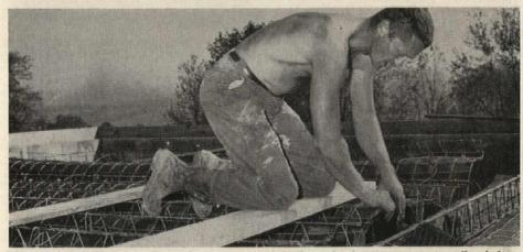
Wire mesh installed at arch openings prevents drip-through of wet concrete to cellar below
