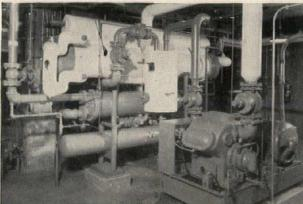
This Vilter air conditioning plant consists of a Freon shell and tube water chiller, shell and tube condenser, liquid receiver and a six-cylinder Freon VMC compressor, all installed in the Southwestern Bell Telephone Co., Olathe, Kansas.
