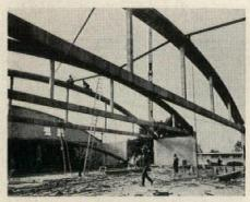
Hundred-foot trusses are lowered onto pilasters spaced 18 ft, 8 in. apart. Four have an arch of 13 ft; four arch 11 ft, giving appearance of folded shell. Each supports a live load of 40 psf
